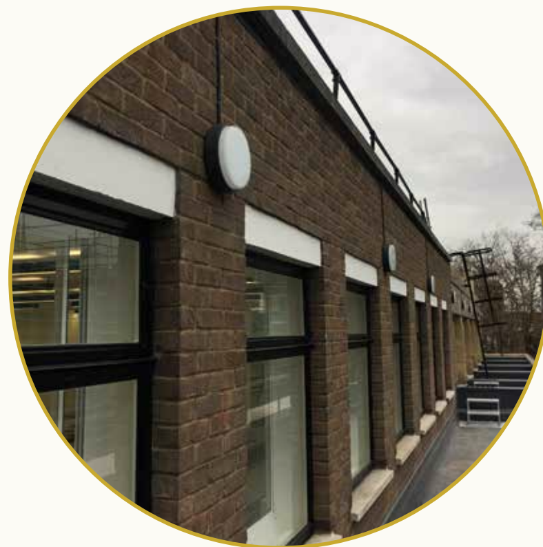
INSTALLED REPLACEMENT LIGHT FITTINGS TO DANE STREET TERRACE.
