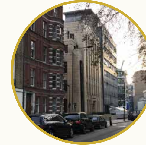
IMAGE 1 VIEW LOOKING SOUTHWEST FROM RED LION SQUARE (SOUTH).
