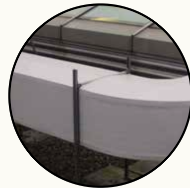
Example of white Ductwork Wrap.
