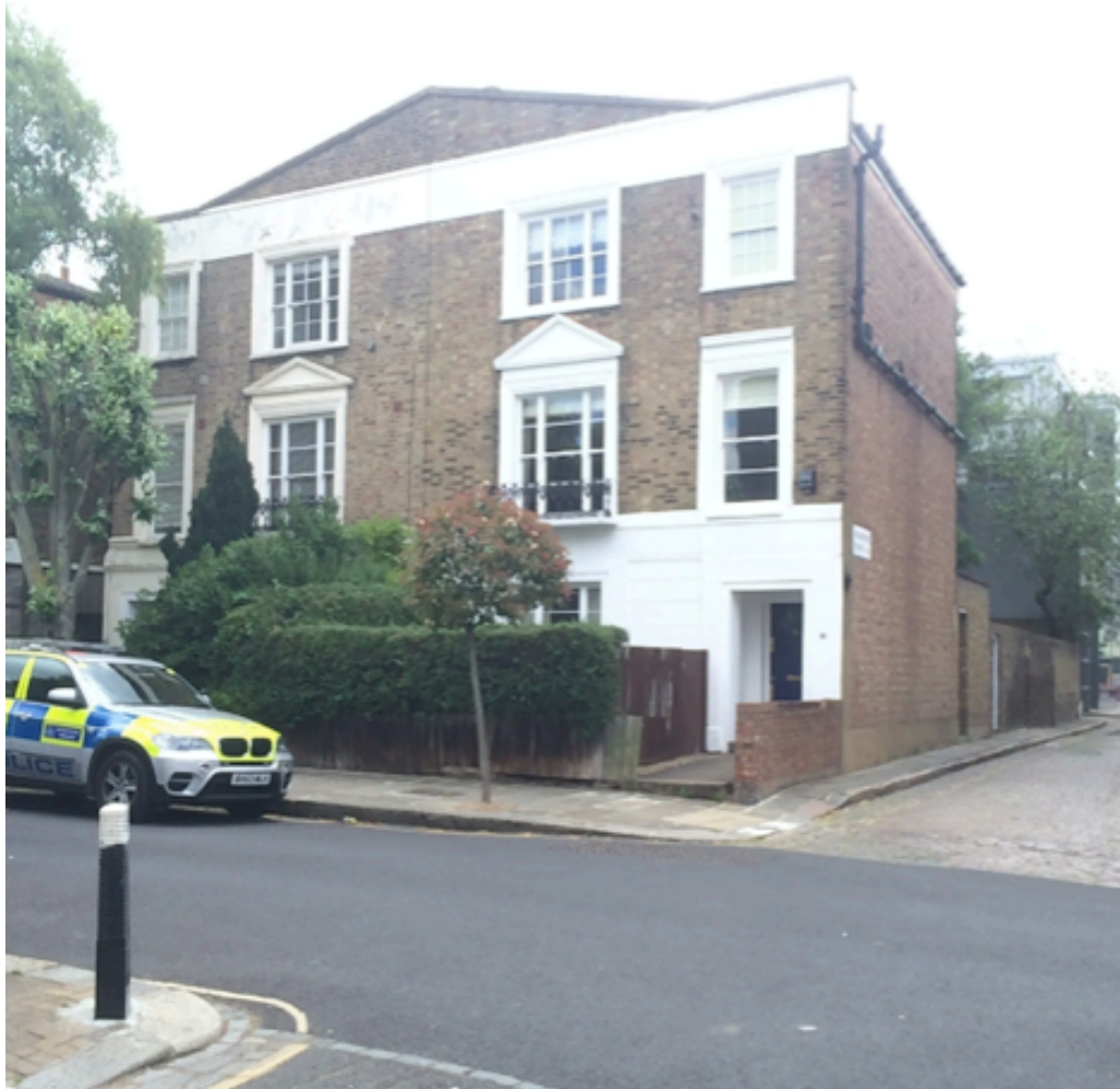
Front view of No. 15 Wilmot Place
