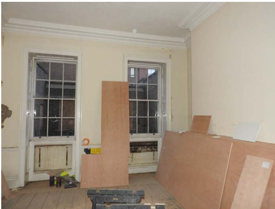
Fig. 7 No 15 lightwell from the rear ground floor room
