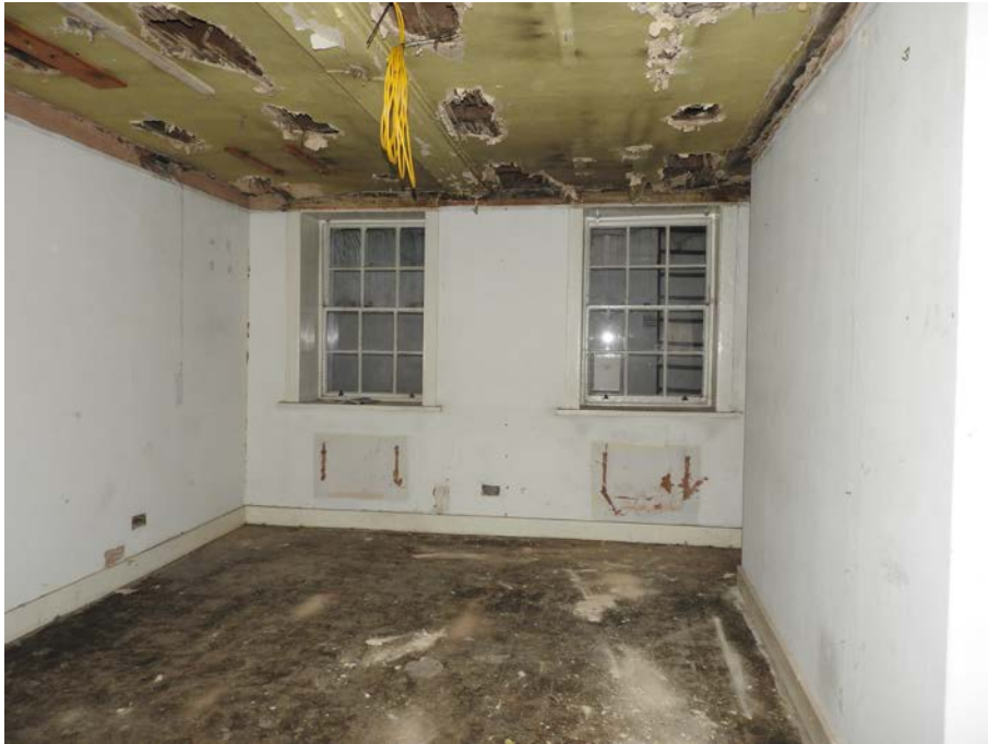
Fig. 8 Lower ground floor rear room where the shower facilities are proposed.
