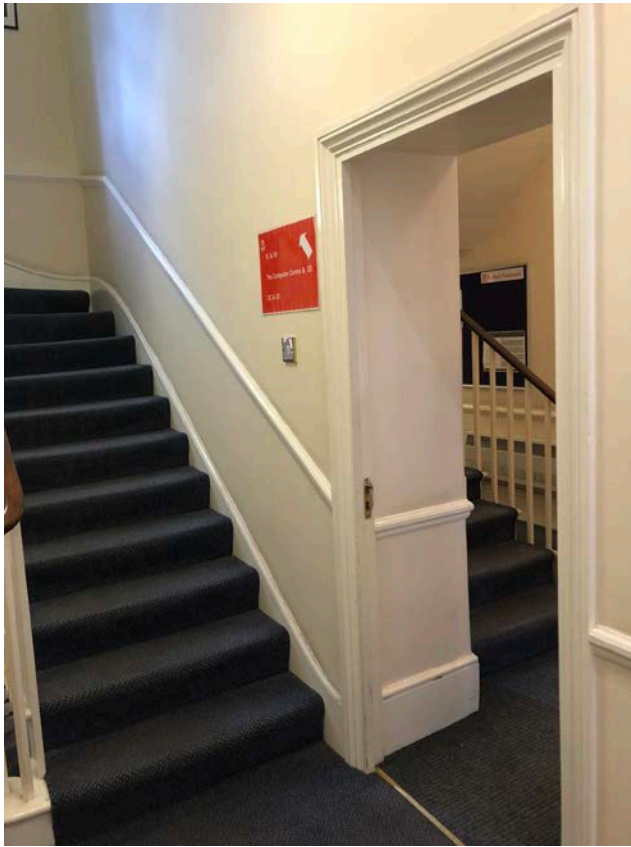
Fig. 6 No 20 and 21 Southampton Place at Ground Floor level.
