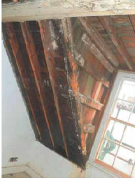
02 DRY ROT TO MANSARD & ROOF CONSTRUCTION IN No. 15
