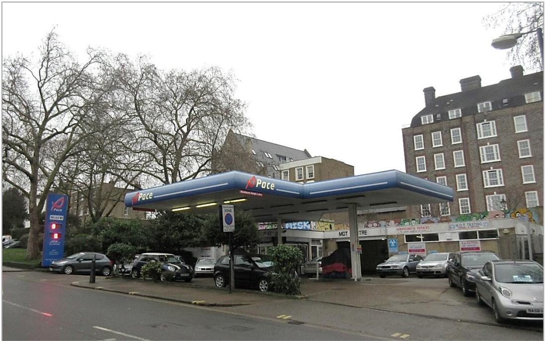
Figure 12: Application site, February 2018
