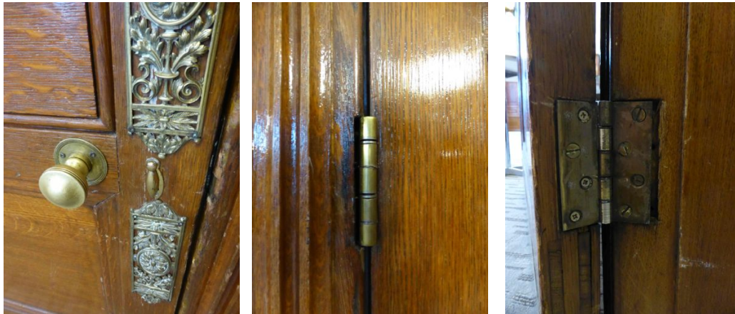
Figs. 6, 7, 8 Boardroom entry door – original handle/push plate / excessively worn hinges / poor fitting in 2012
