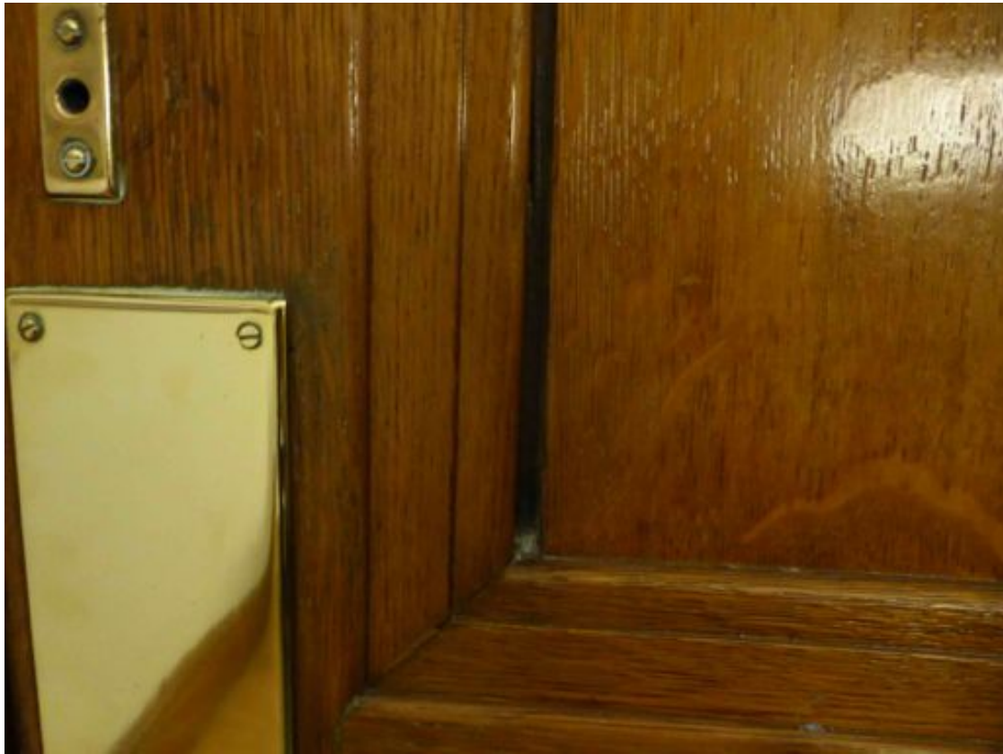
Fig. 24 Split in upper panel left edge requiring oak spliced repair
