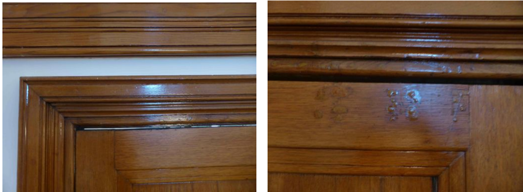
Figs. 11, 12 Oak entry door, gap to frame head / door closer repair
