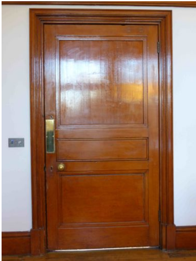
Figs. 9, 10 Oak entry door inner face, original colour of doorframe - Note gap under door re. Part B fire regulations - relatively recent hinges in plated steel
