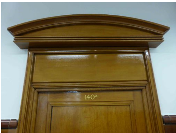
Fig. 13 Oak pediment common to minor boardroom doors – distinct colour difference to the interior
