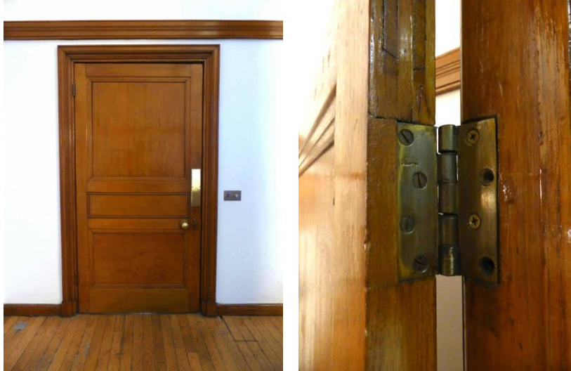
Fig. 25 26 Oak entry door with original ironmongery – hinge with evidence of replacement
