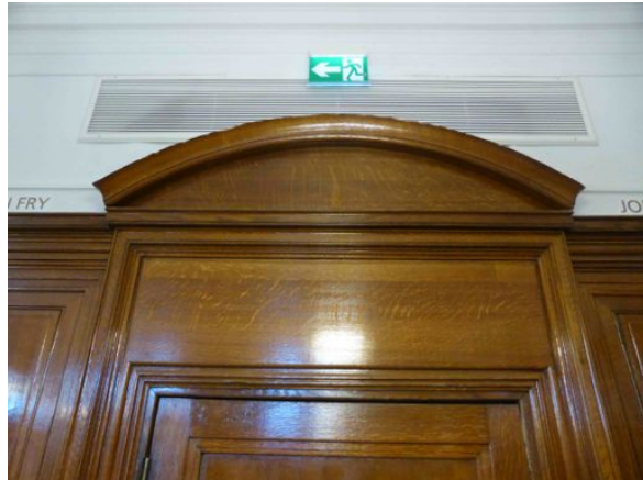
Figs. 3, 4 Boardroom entry door – high gloss varnish / pedimented head with friable edge – AC grille above
