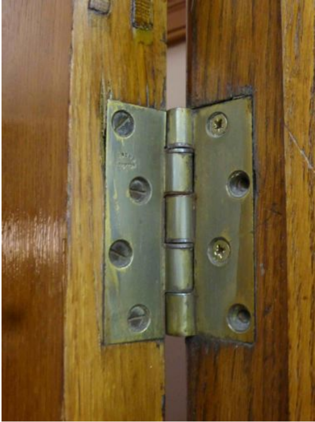
Fig. 19 Hinge detail to door – modern washed hinge showing wear
