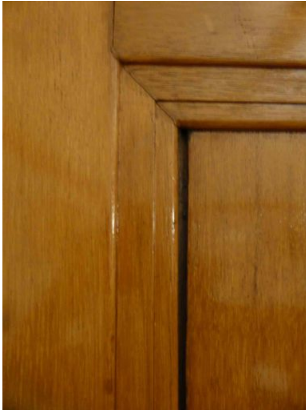
Fig. 28 Oak splice required for upper panel edge on the inside face
