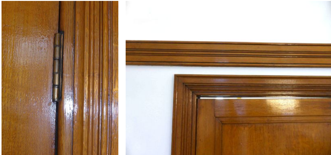
Fig. 20 21 Oak entry door – significantly worn hinges - unacceptable gap for fire safety
