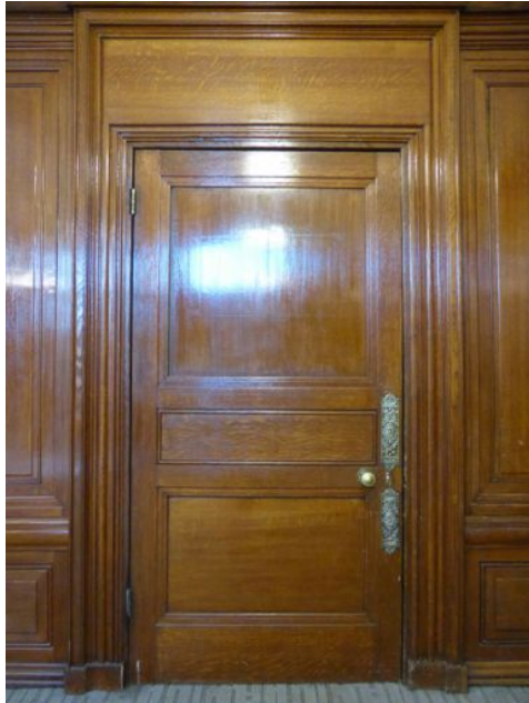
Figs. 3, 4 Boardroom entry door – high gloss varnish / pedimented head with friable edge – AC grille above
