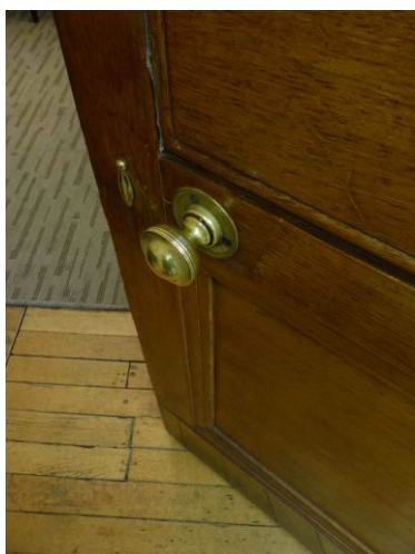
Figs. 17, 18 Original door with original ironmongery, gap to frame in breach of fire safety requirements
