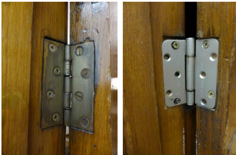
Fig. 22 23 Older hinge but poor fit shows unoriginality, modern replacement without consideration
