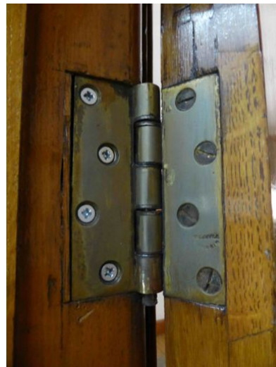
Figs. 9, 10 Oak entry door inner face, original colour of doorframe - Note gap under door re. Part B fire regulations - relatively recent hinges in plated steel
