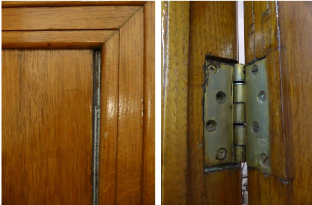
Figs. 14 , 15 Oak panel requiring splicing in – plated steel washered hinge worn and a poor fit
