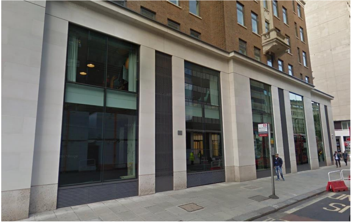
Photo of the South Elevation Louvres located on the ground floor (New Oxford Street)
