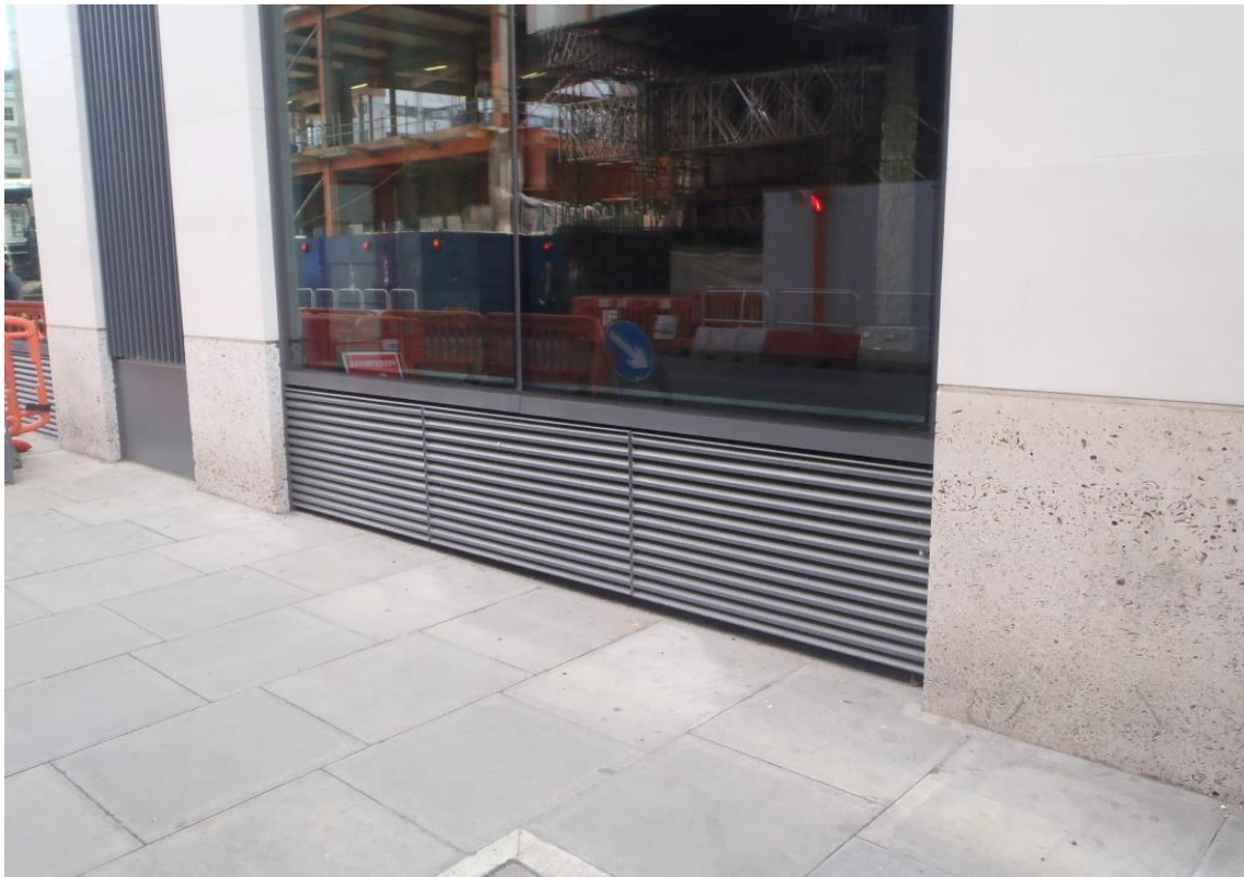
Photo of the South Elevation Louvres located on the ground floor (New Oxford Street)
