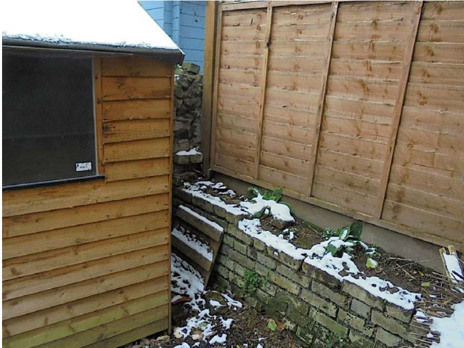
Photograph 7 – Retaining wall adjacent to T4
