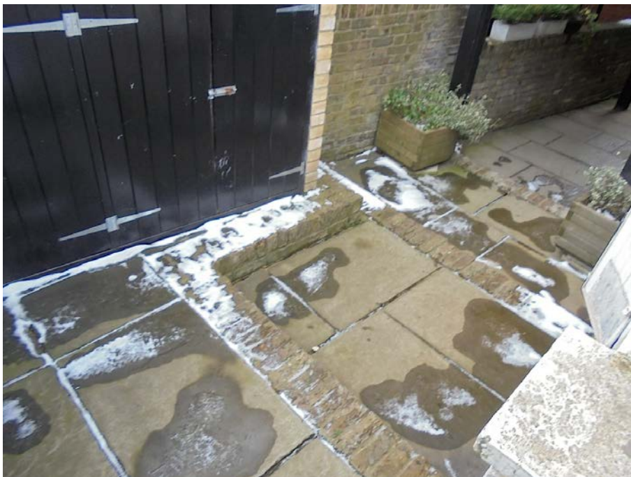
Photograph 4 – Hard standing within root protection area of T5
