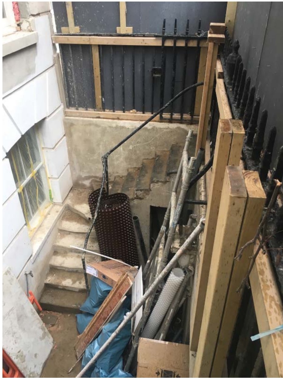
01. No. 67 Previously existing balustrade
