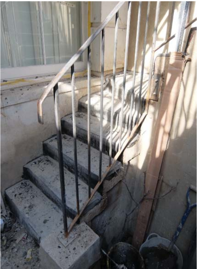
07. No. 67 new balustrade
