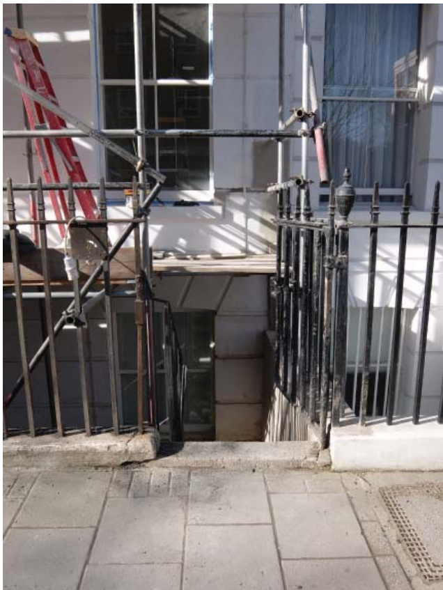
02. No. 67 new balustrade
