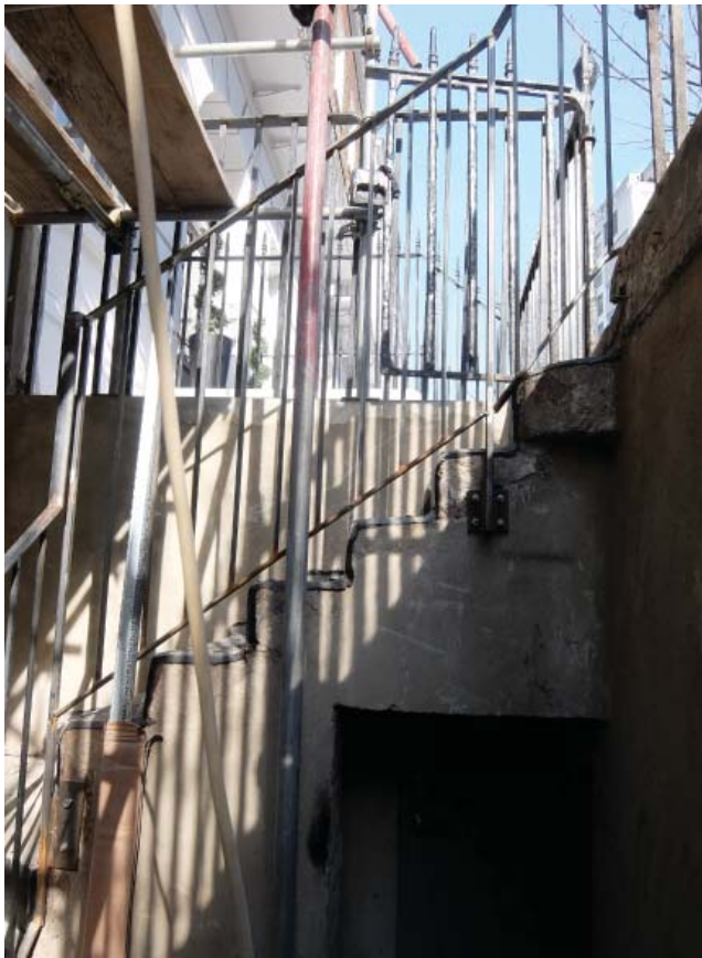
05. No. 67 new balustrade
