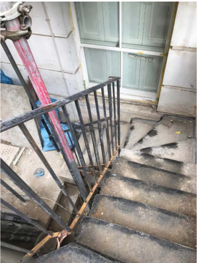
04. No. 67 new balustrade
