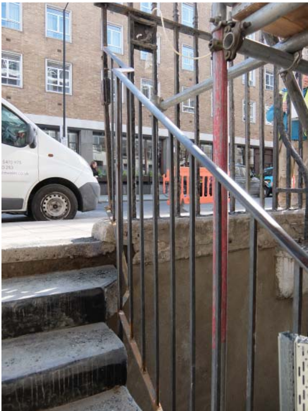
03. No. 67 new balustrade
