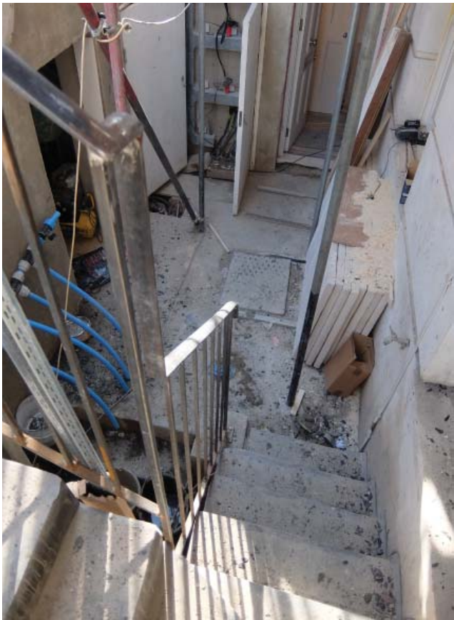
06. No. 67 new balustrade
