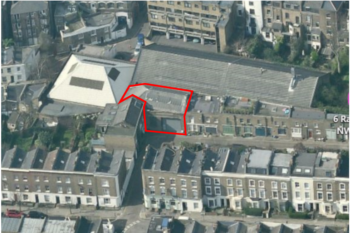
4) Aerial image of site outlined in red
