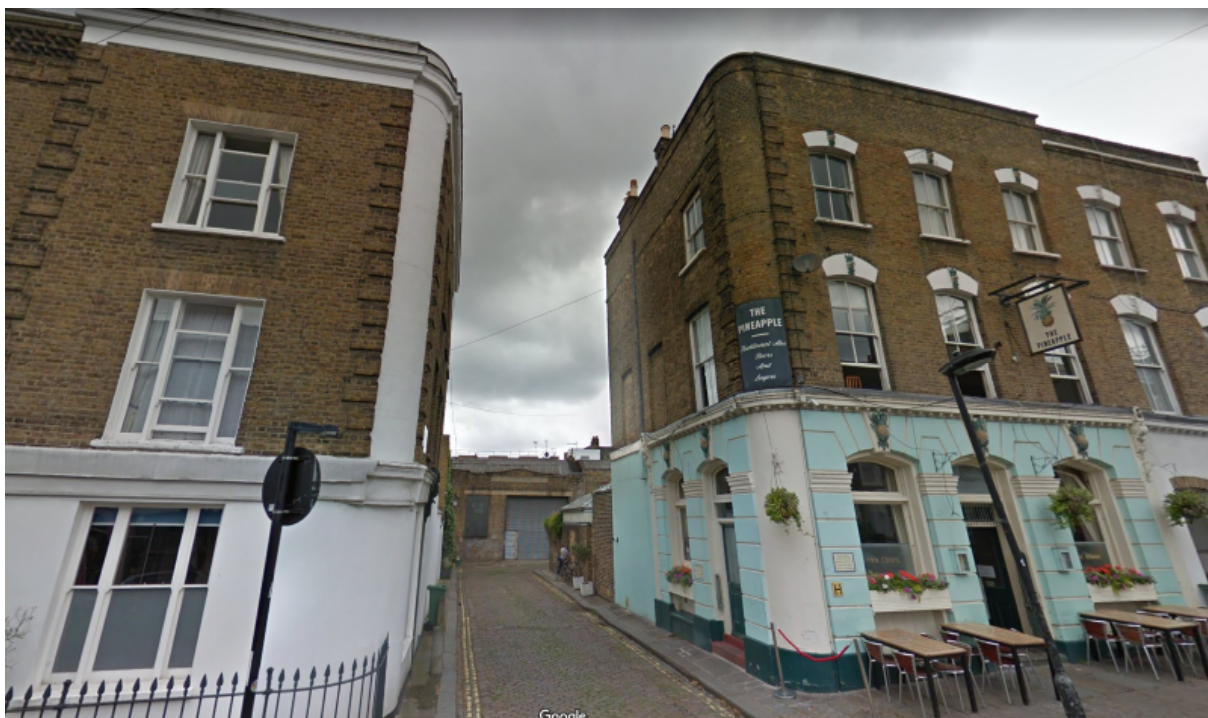
3) Long view of site down Railey Mews, The Pineapple (Grade II Listed pub) in foreground
