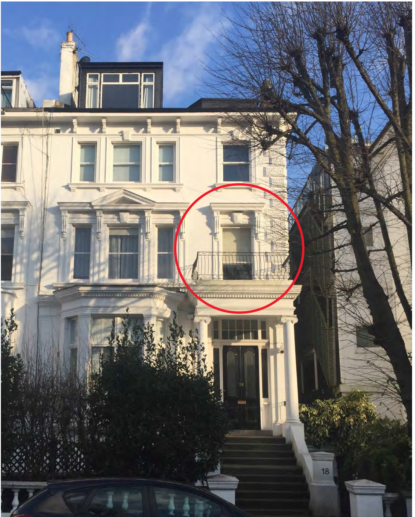
18 Belsize Grove: view of the existing sash window exit to existing balcony from outside.
