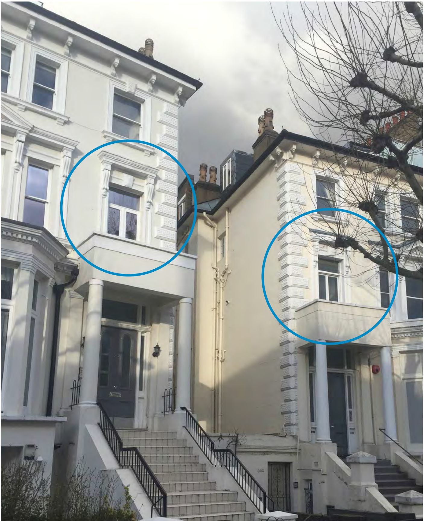
Examples of existing french doors and fixed panel above (matching our proposal) found in close proximity of the site: No. 52 & 54 Belsize Park Gardens.
