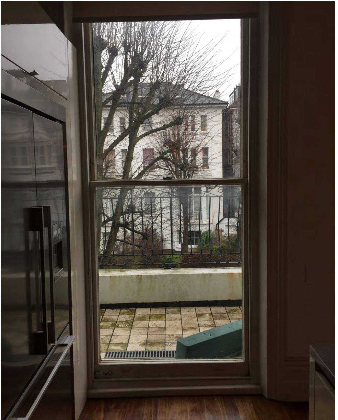
18 Belsize Grove: view of existing sash window exit to existing balcony from inside (kitchen area).
