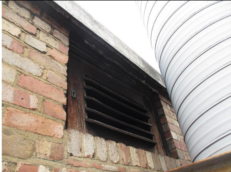
Photograph 7 Louvered door into lift overrun without grill
