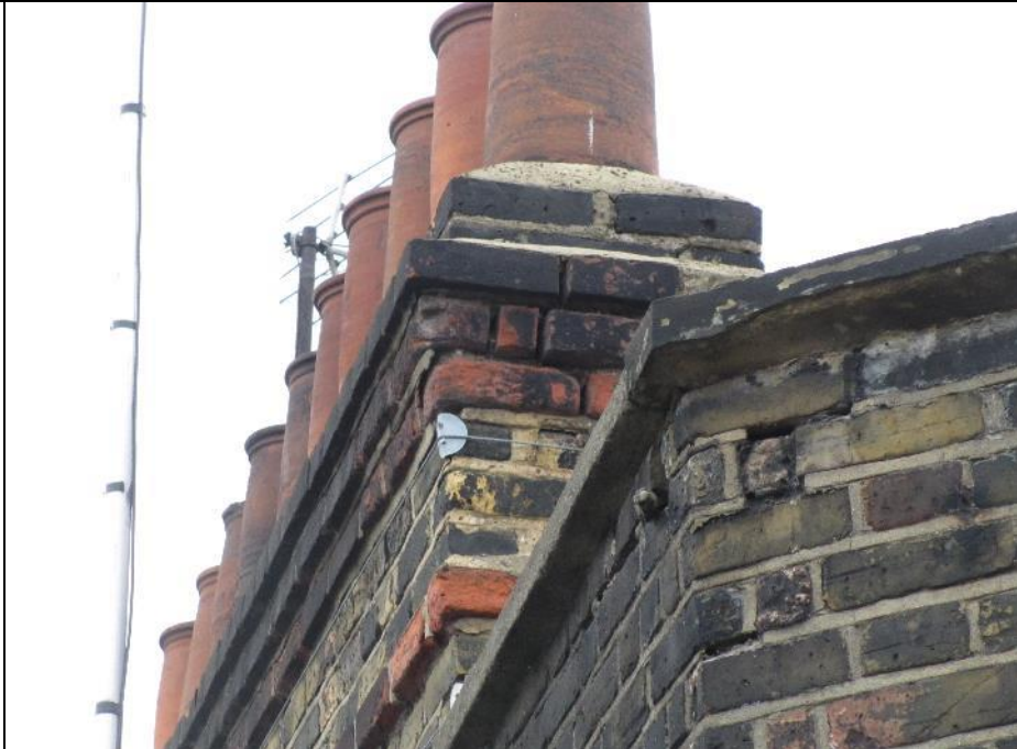
Photograph 9 Missing mortar on adjacent building overlooking the site
