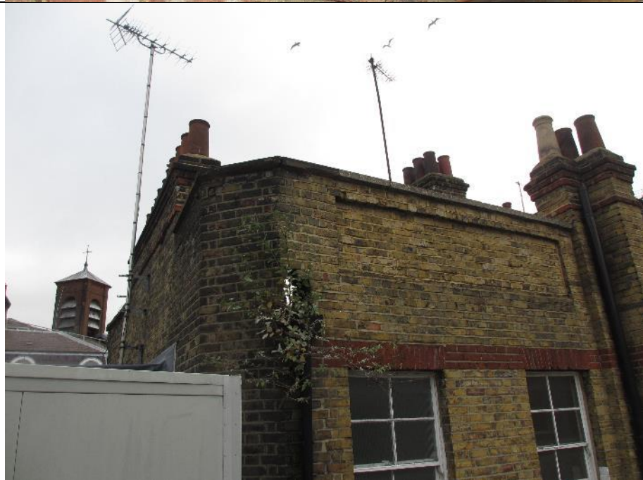
Photograph 8 Adjacent building with butterfly bush and missing mortar on façade overlooking the site
