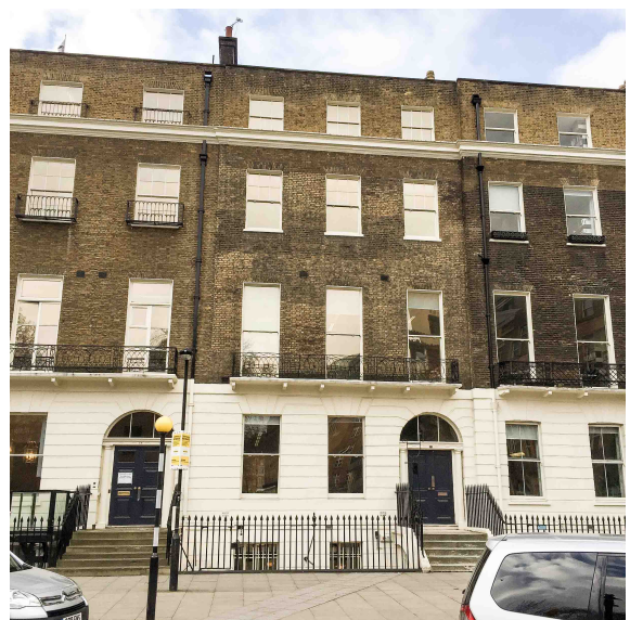
Image 1, View of Front Facade.
