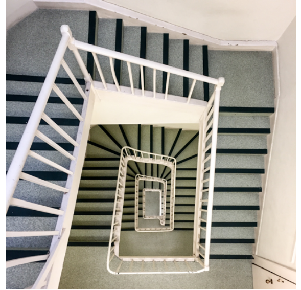
Image 4, View of Rear Staircase
