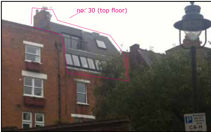
Photo below: showing existing balcony door, October 2014 No.30 top floor flat
