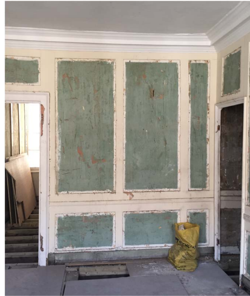
700_601 05 Example of existing timber panelling in good condition Bedroom II r2.03
