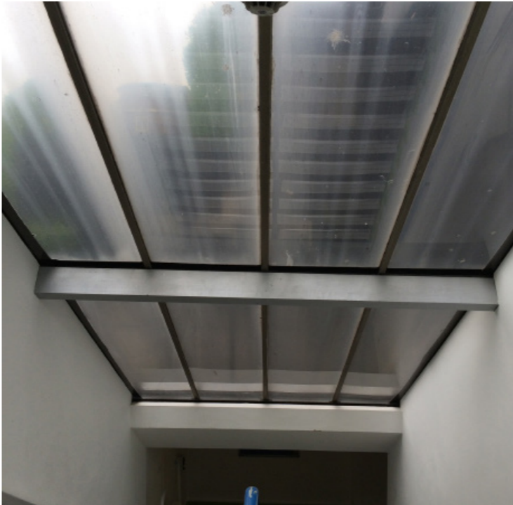
Wired glass rooflights above Stairs Level 3 wing to be replaced
