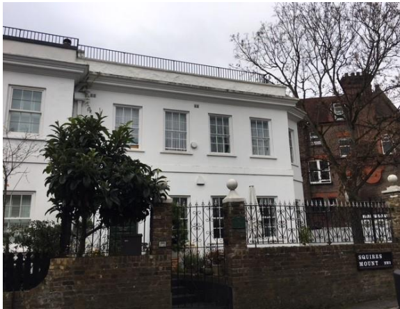
Front elevation showing existing roof terrace across entire building (top) and adjoining neighbour (no. 11)
