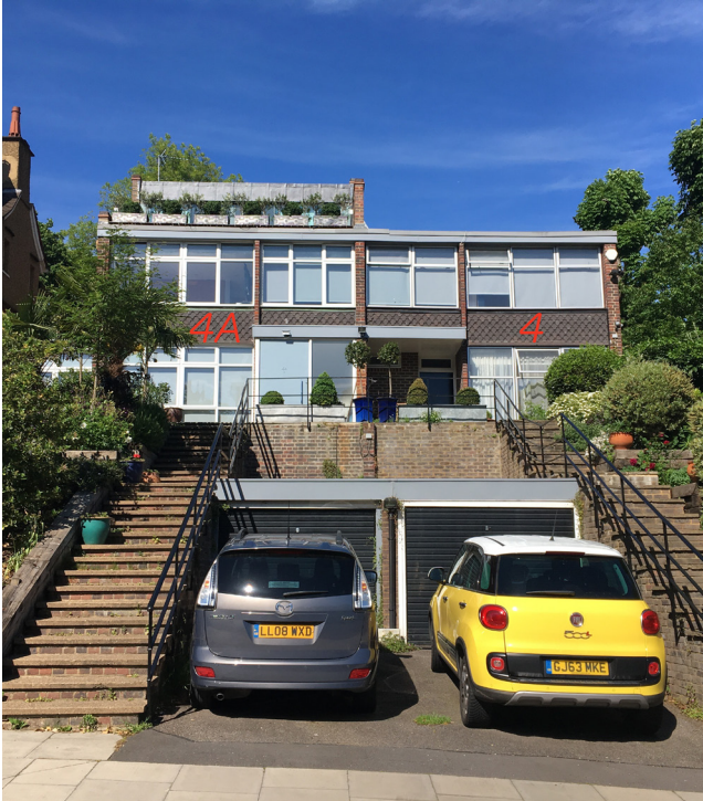
View of n. 4 and 4a front elevation from Lindfield Gardens.
