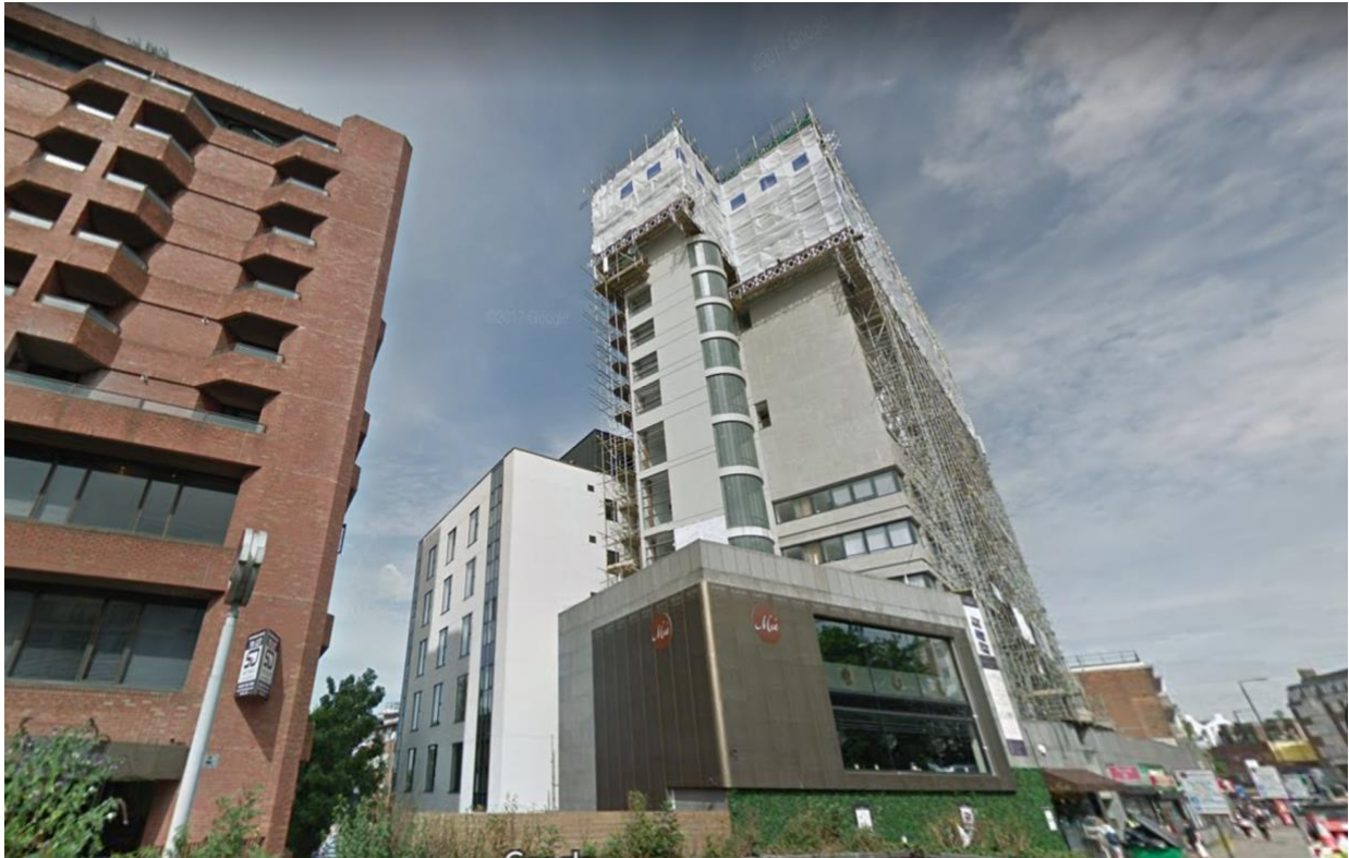
Photograph 2 – 135 Finchley Road –Perforated Aluminium cladding installed
