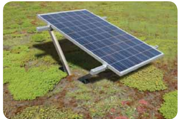
Mounted photovoltaic panel prior to the installation of the ballasting green roof and vegetation.
