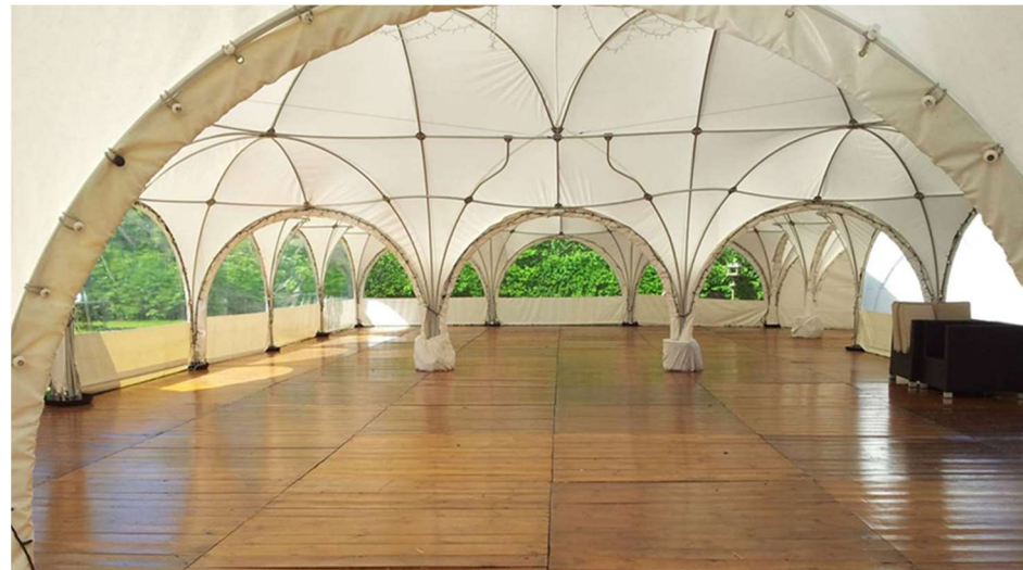
Photo of the inside of the marquee, showing fixture to wooden flooring
