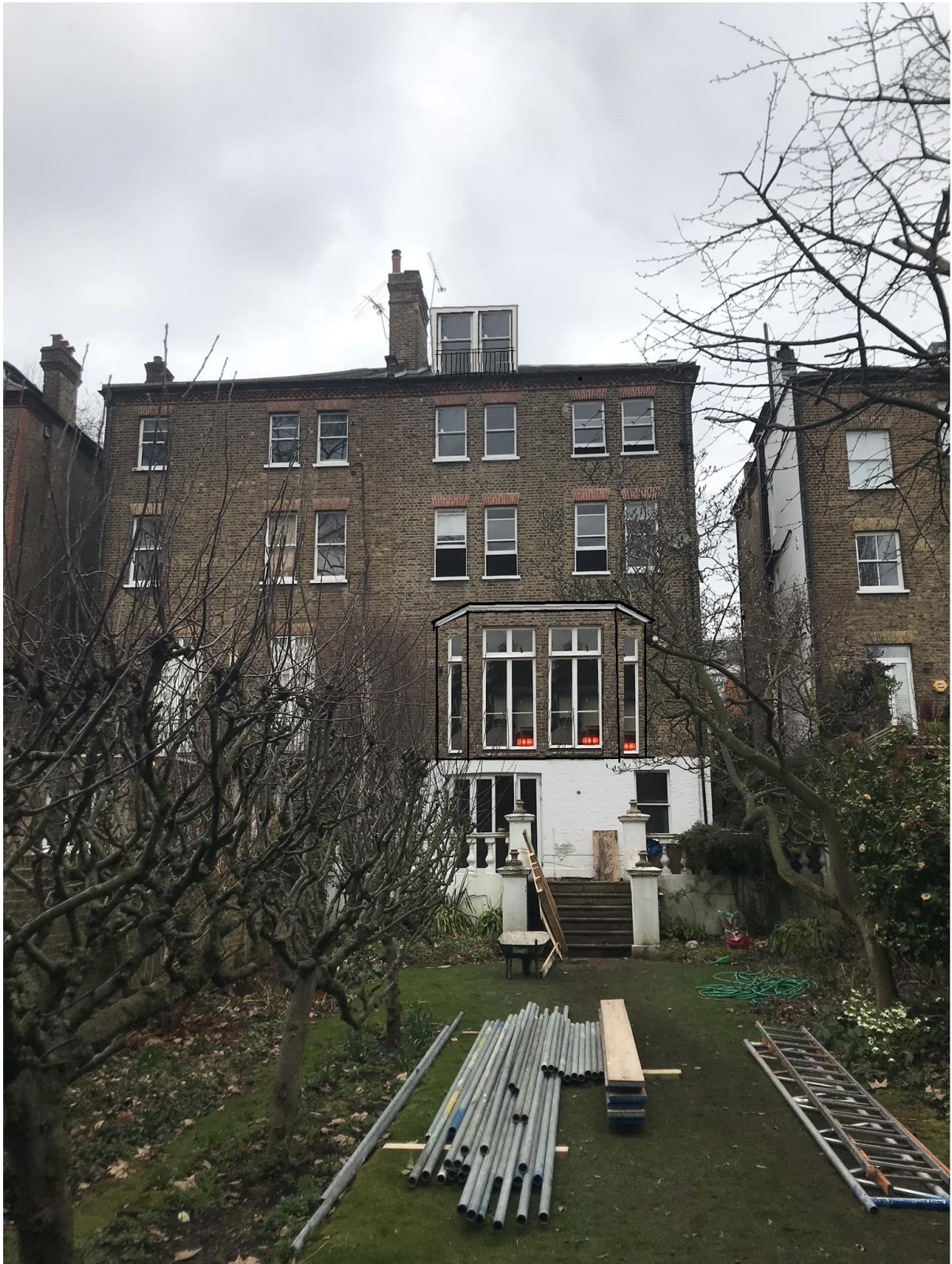
PHOTOMONTAGE SHOWING PROPOSED AMENDMENTS. JULIET BACONY TO REAR DORMER WINDOW, ADDITIONAL SASH WINDOWS TO FIRST AND SECOND FLOOR AND BAY WINDOW TO GROUND FLOOR
