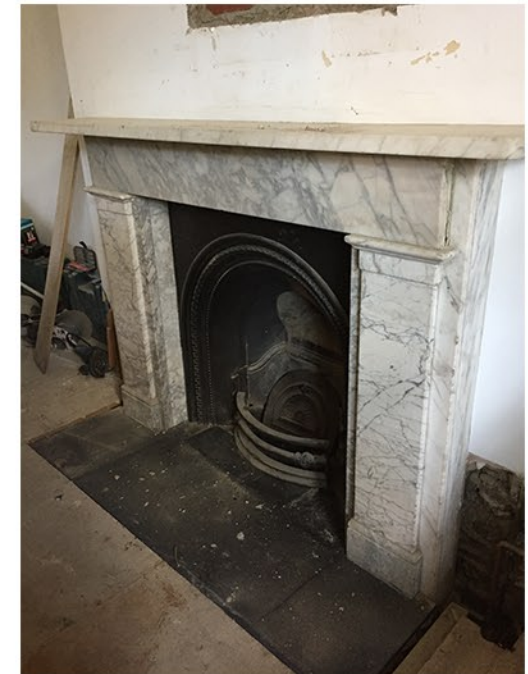
LIVING ROOM Retain and repair existing original Victorian carrara marble fireplace surround with original arched cast iron fire insert operating on gas fire
