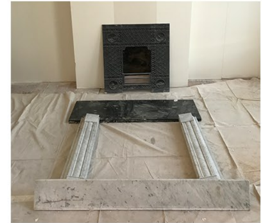
DRESSING ROOM Original Regency carrara marble fireplace surround with original rectangular cast iron fire insert decorative feature only
