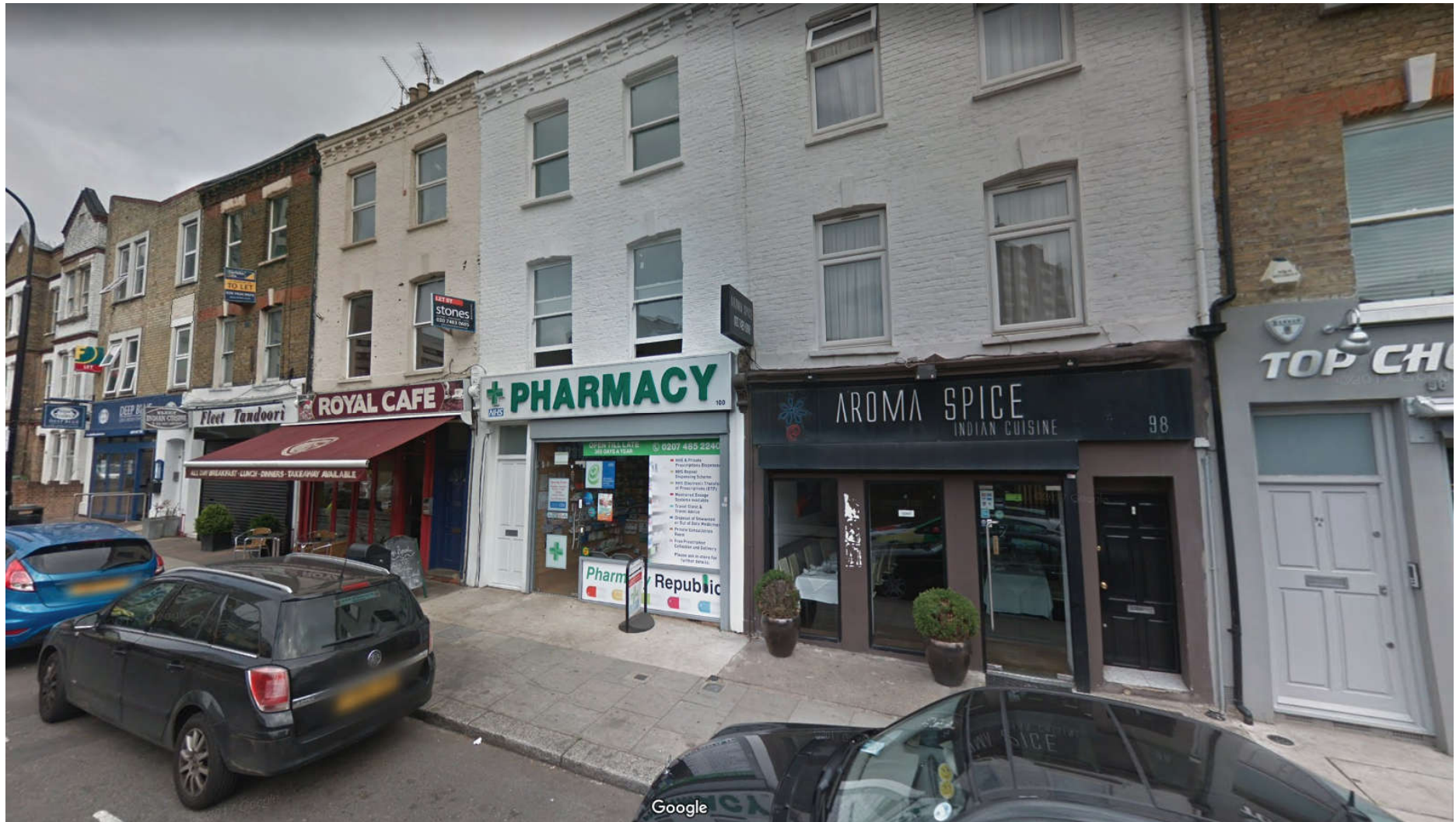
View of additional shopfronts to the north west (Source: Google)
