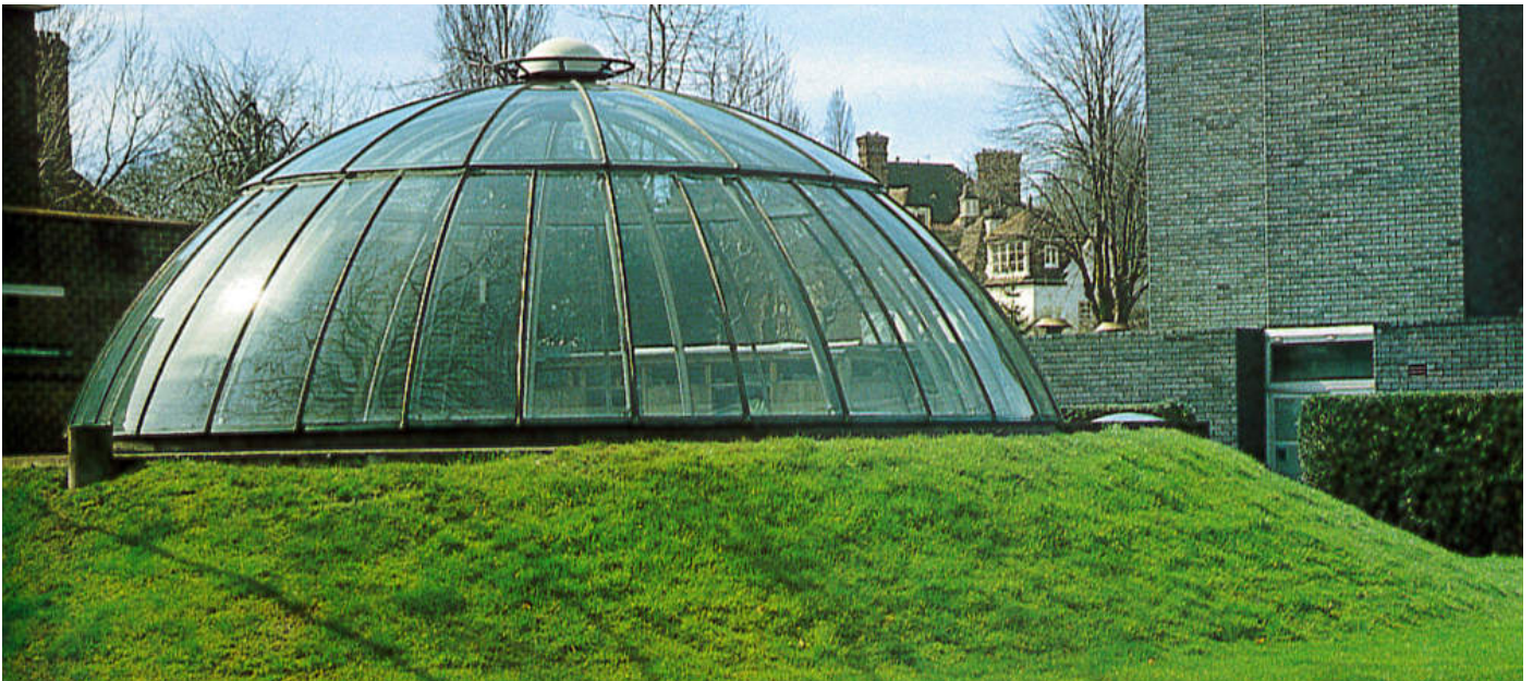
20. Exterior view of the pool building
