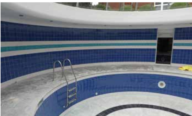
7. Interior view of the pool
