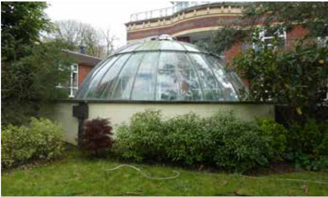
1. Exterior view of the pool building
