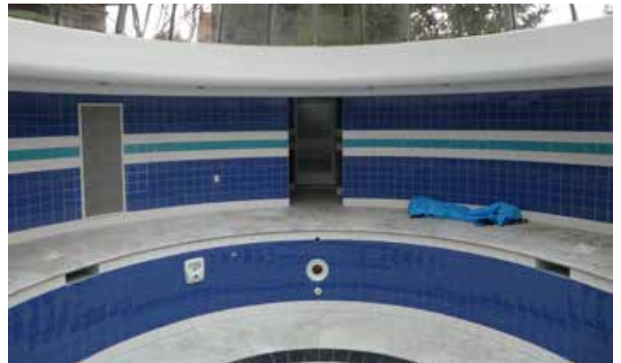
6. Interior view of the pool
