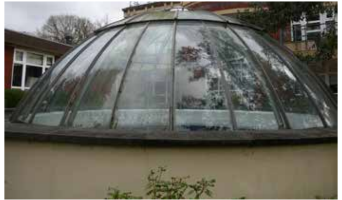
4. Exterior view of the glazed dome
