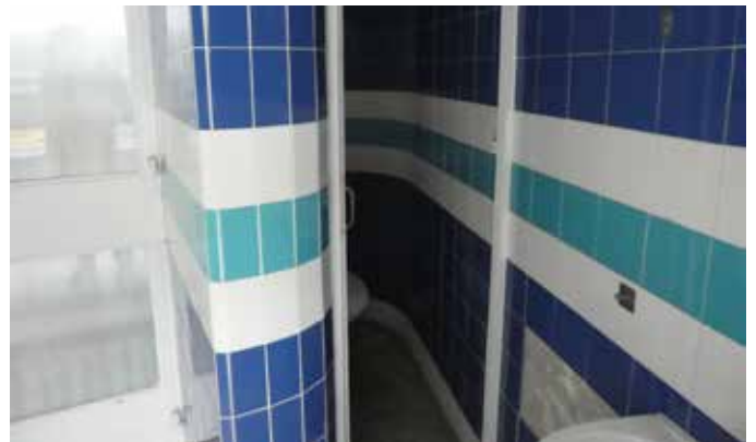
12. Interior view of the WC
