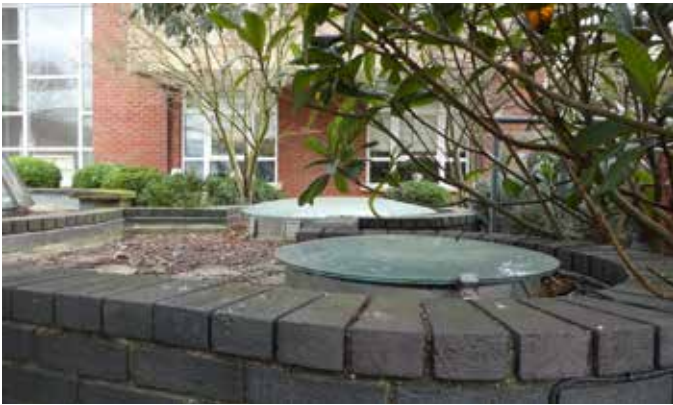
3. View of skylights over shower and WC
