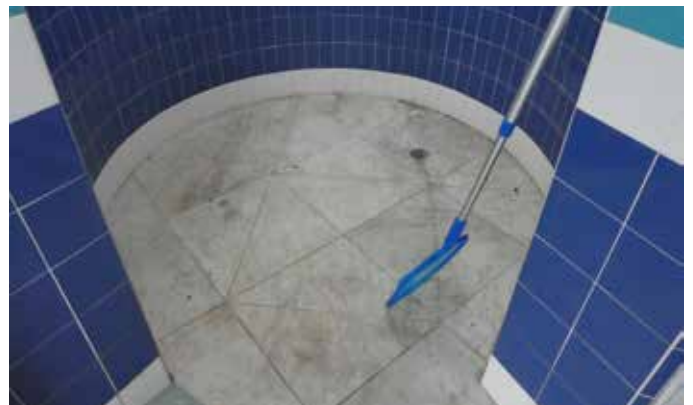
14. Interior view of the marble floor to the shower area
