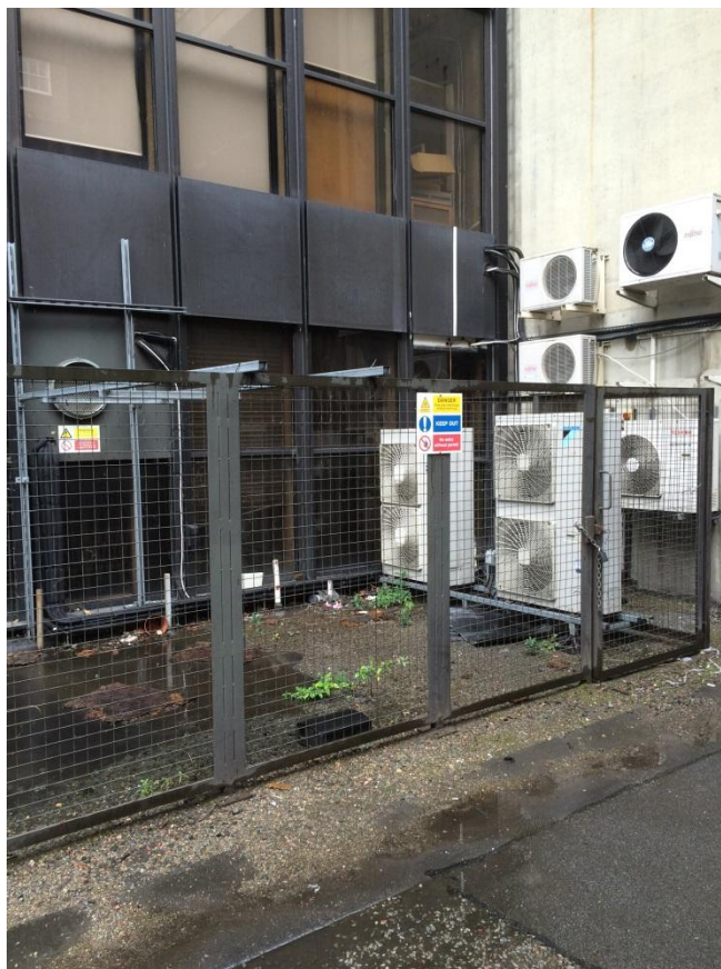
Figure 2 - Rooms B21 & B23 as Viewed from Rear of Bedford Way
