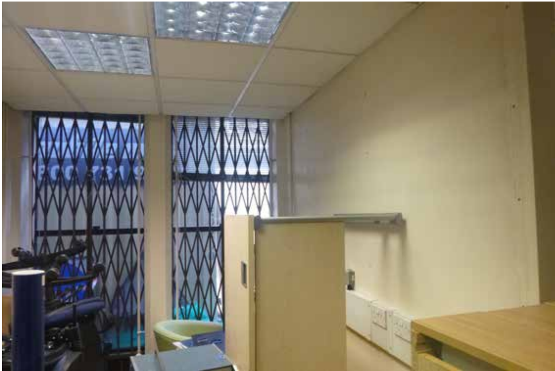
Existing electronics office and stud wall
