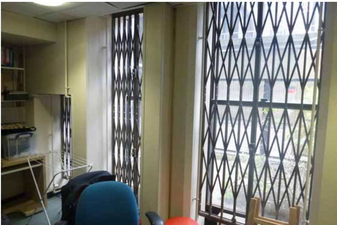
Window detail in existing engineering office
