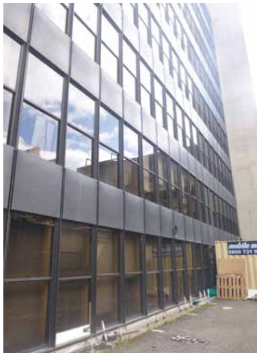
Exterior of the Site, viewed from the service road
