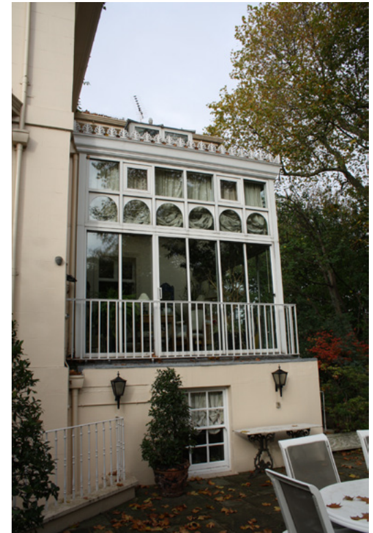
The southern elevation of the conservatory
