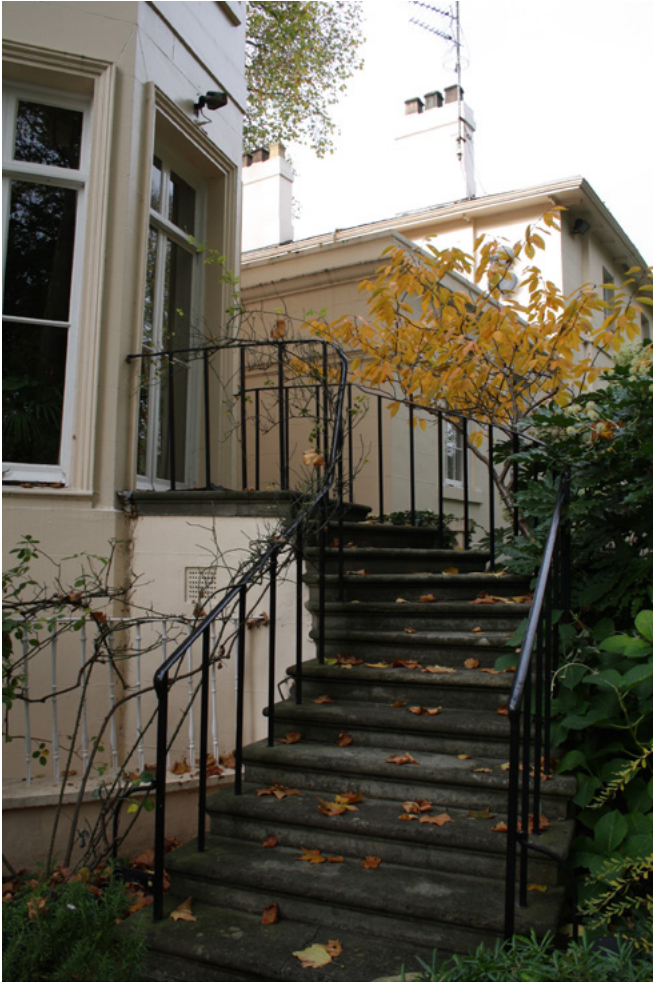
Staircase leading from reception room into the garden on the east elevation
