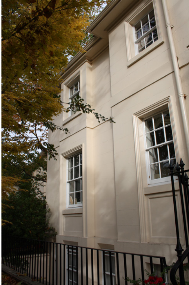
Northern end of principal elevation
