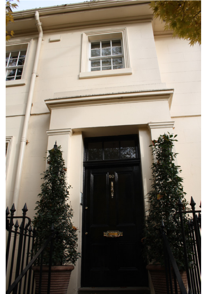
Main entrance door, with plastered surround and accessed via steps
