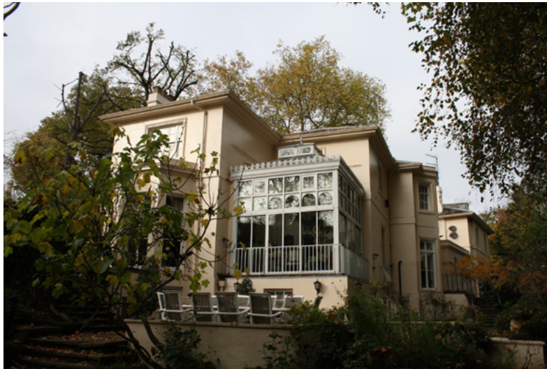
South elevation of the house from the garden
