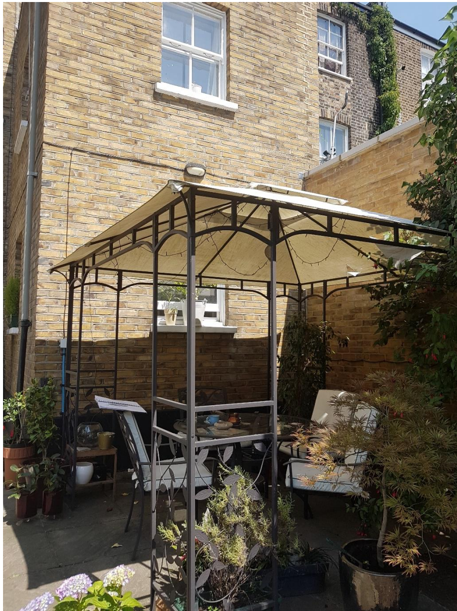
Fig. 2 – Rear of 38A Iverson Road - Right hand side massive wall and extension
