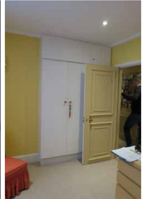
Fitted joinery to be removed
