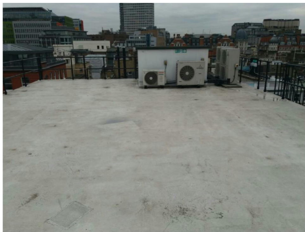
Photographs 1 - Existing Roof
