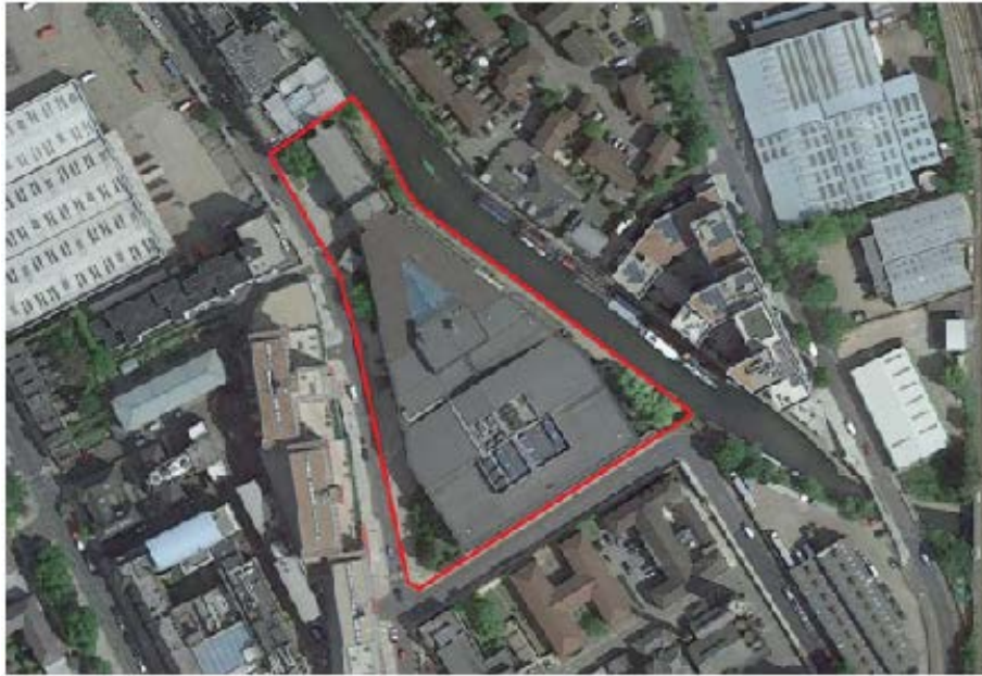
Photo 1: The existing site
