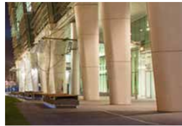
LT1 WALL FIXED OR COLUMN LIGHT
