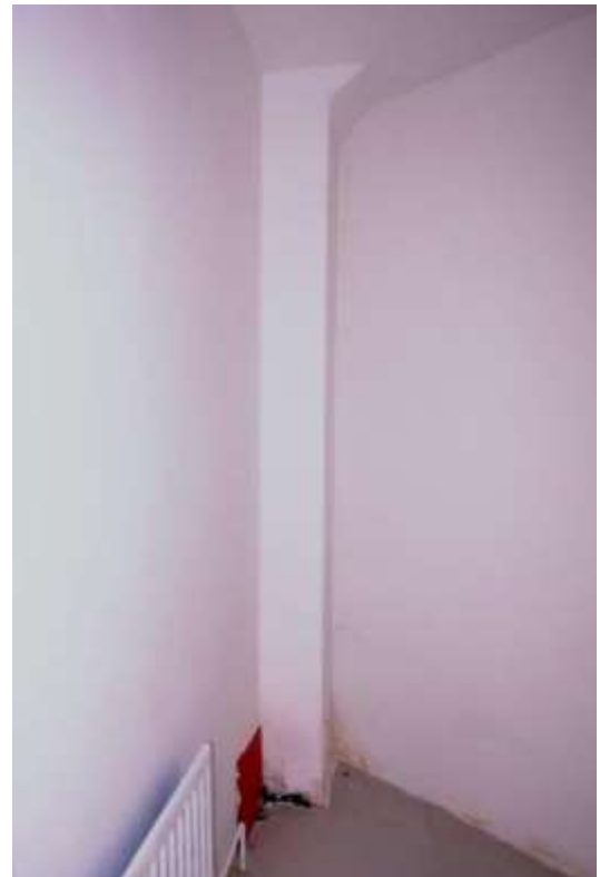
Fig 42 The damp ingress at the bottom of the north-east pier in the south-east room of the basement
