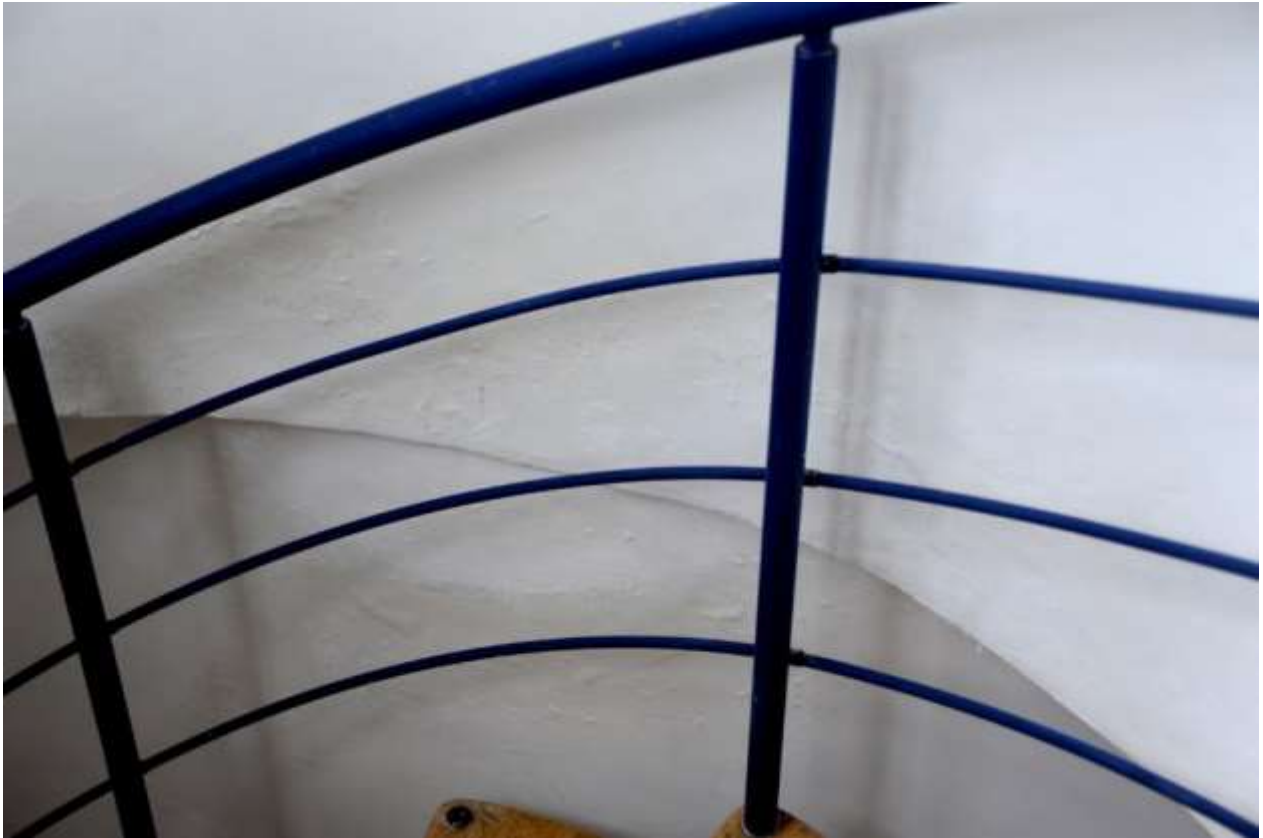
Fig 38 The wall affected by damp at ground floor level in the north-west tower
