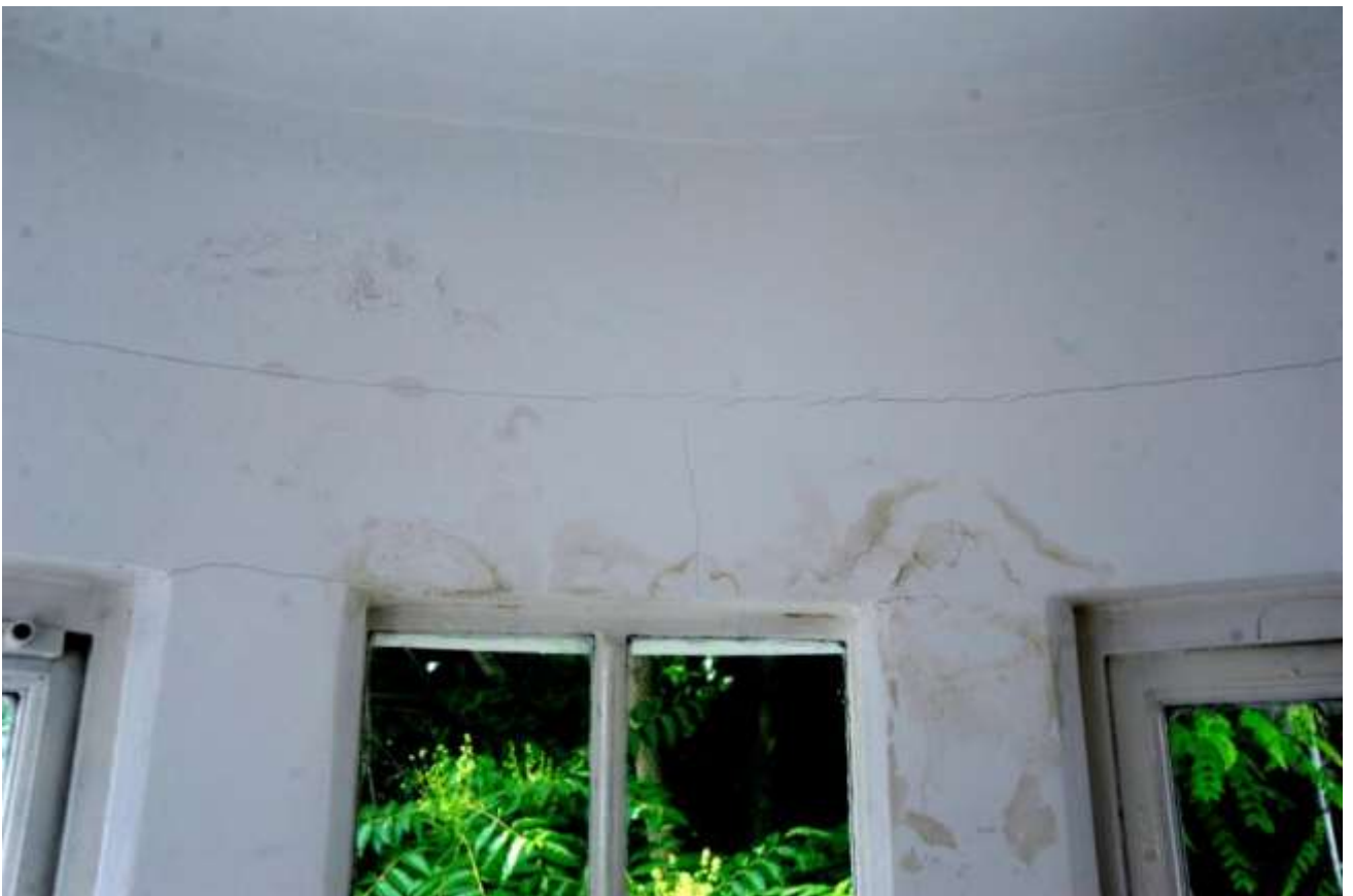
Fig 29 Damp staining above window W50
