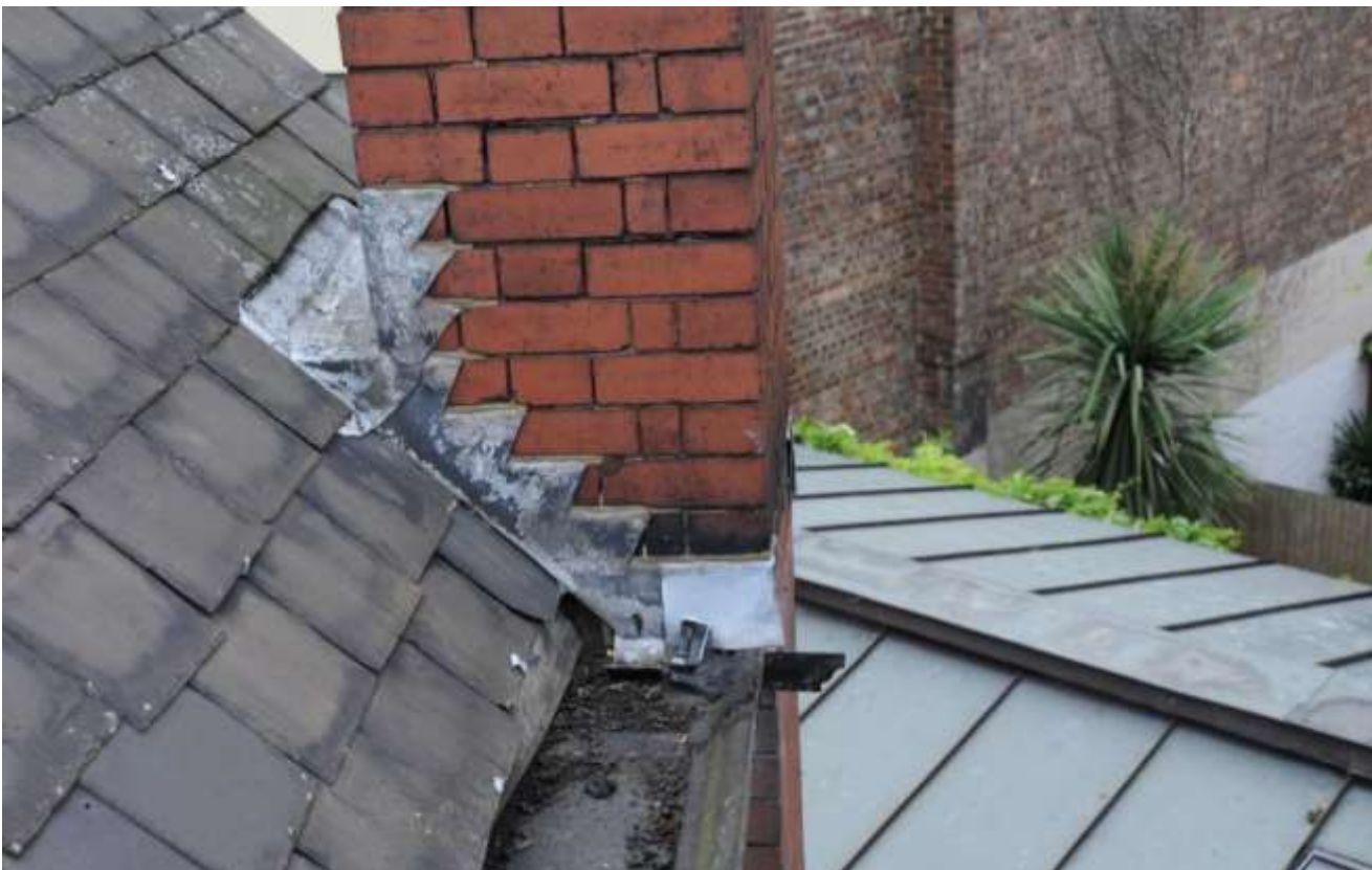
Fig 9 The cast iron gutter and lead flashings at the base of the east chimney stack
