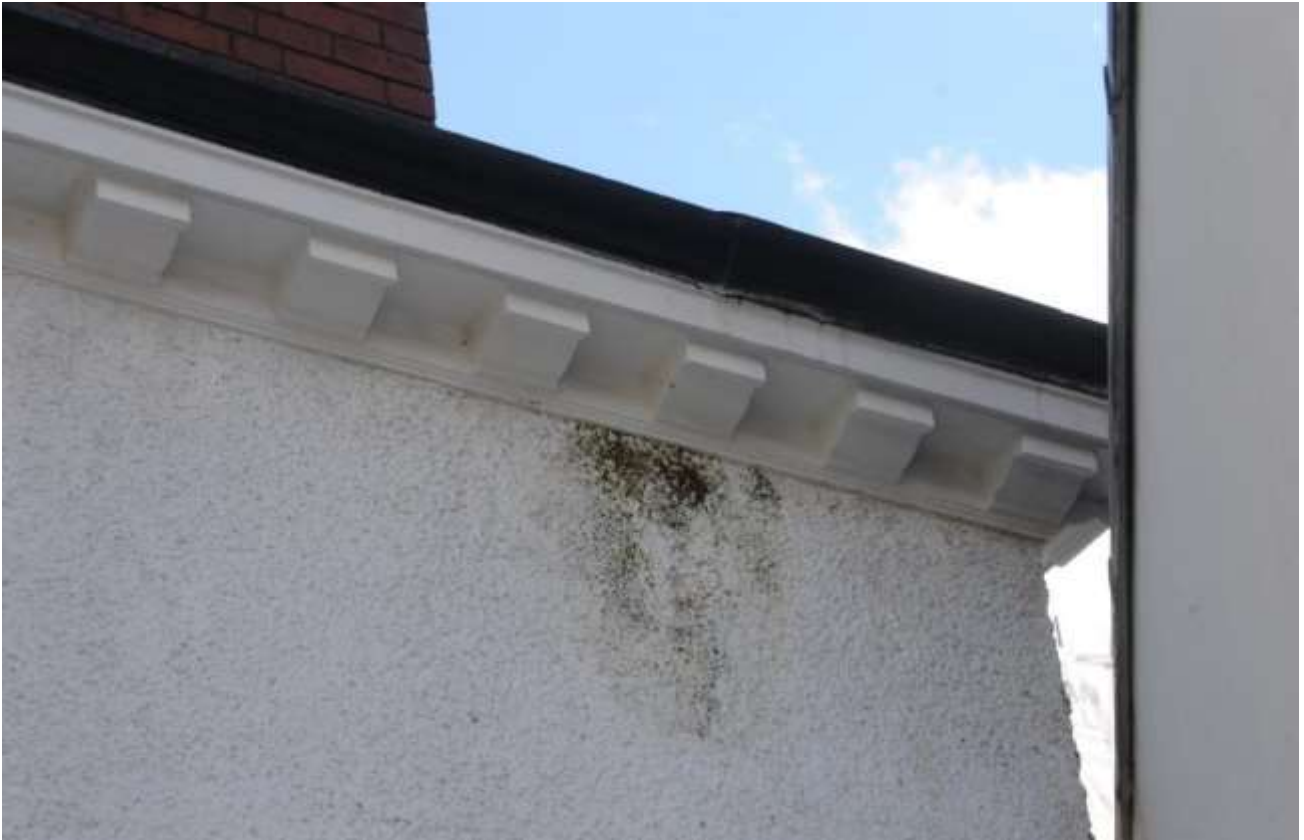
Fig 10 Algae staining of the render under a defective gutter on the south elevation
