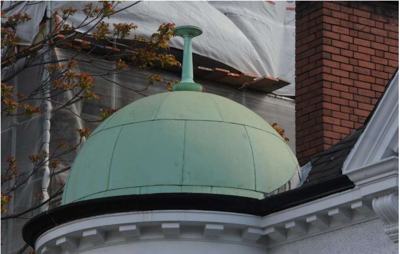
Fig 8 The copper dome over the north-west tower
