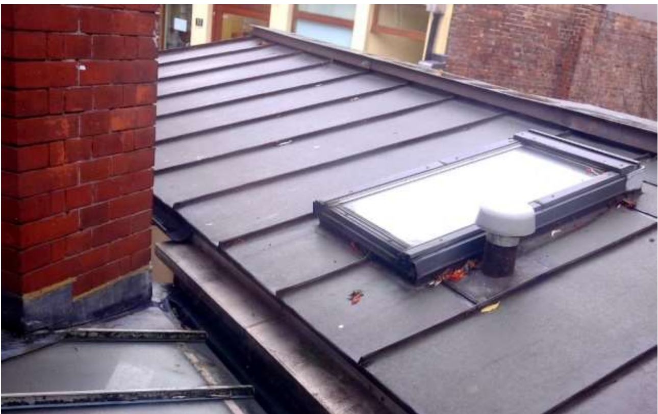
Fig 37 The gutter detail between the east wall of The Lodge and the adjacent property
