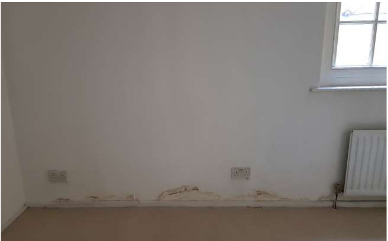
Fig 55 The damp on the west wall
