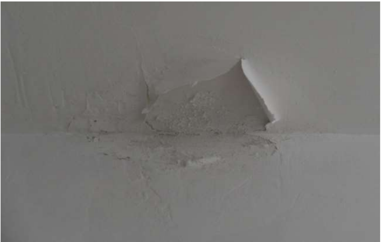
Fig 24 The damp ingress on the ceiling and south wall of the passage in the basement
