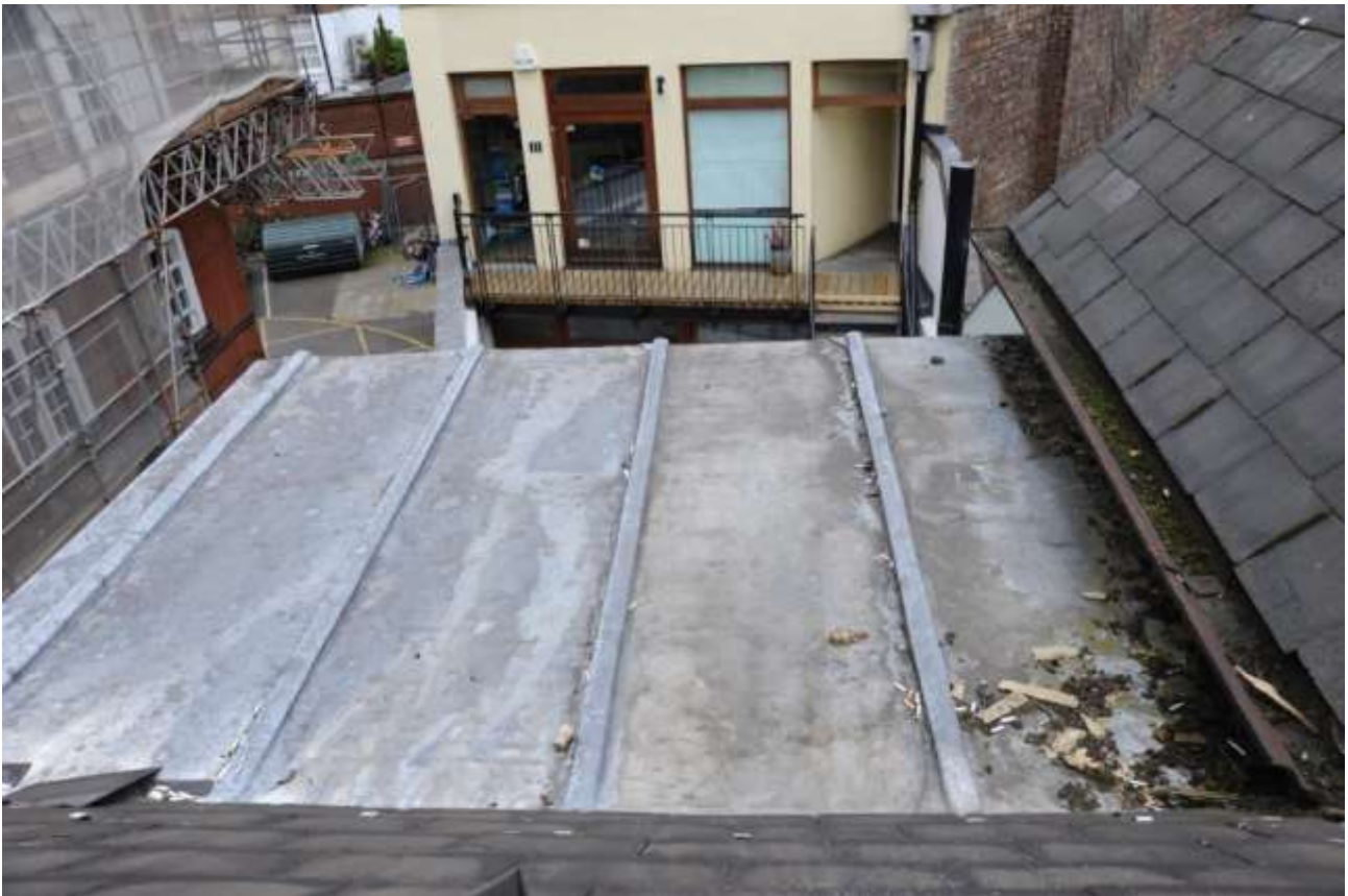
Fig 7 The lead roof over the rear dormer
