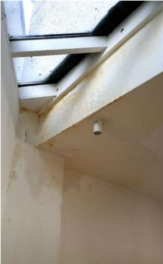
Fig 53 The damp at the south end of the glazed roof on the ground floor.
