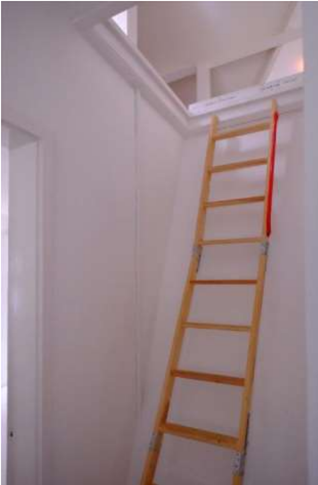
Fig 46 The loft ladder and attic access hatch
