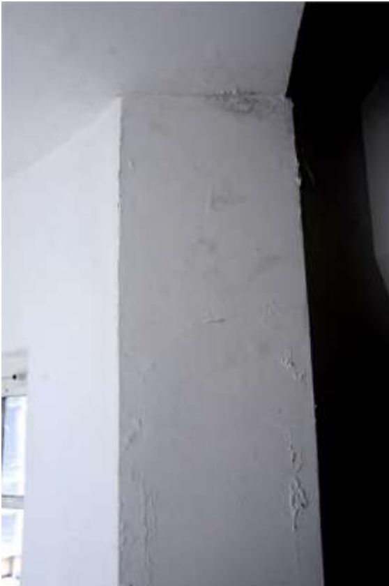
Fig 30 The damp ingress on the wall at the transition between the north-west tower and north room on the first floor
