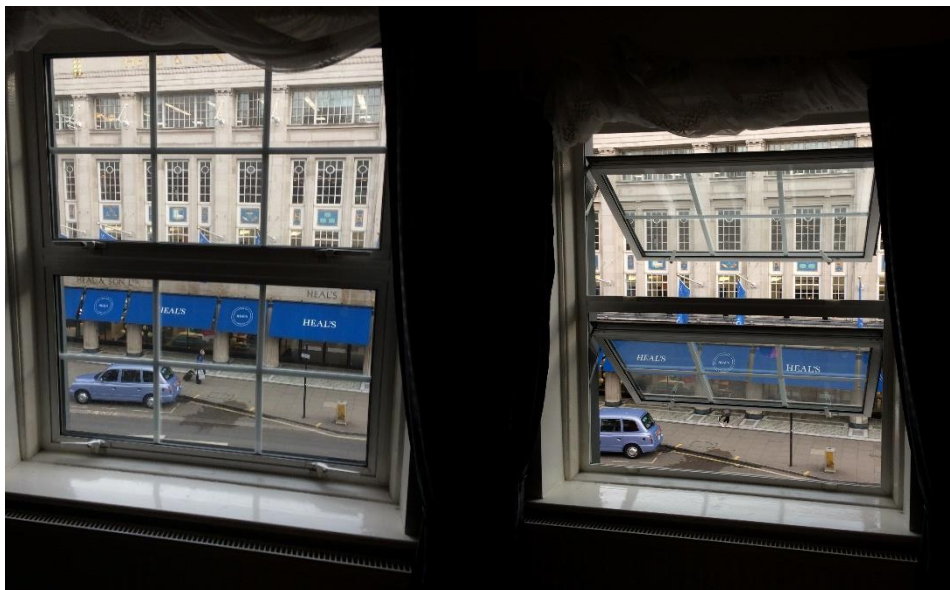
Above: Existing aluminium casement windows at the Property
