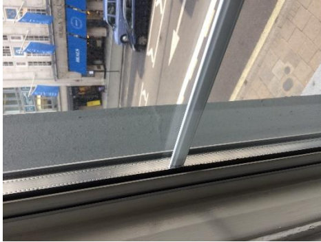
Above: Existing internal Georgian bars
