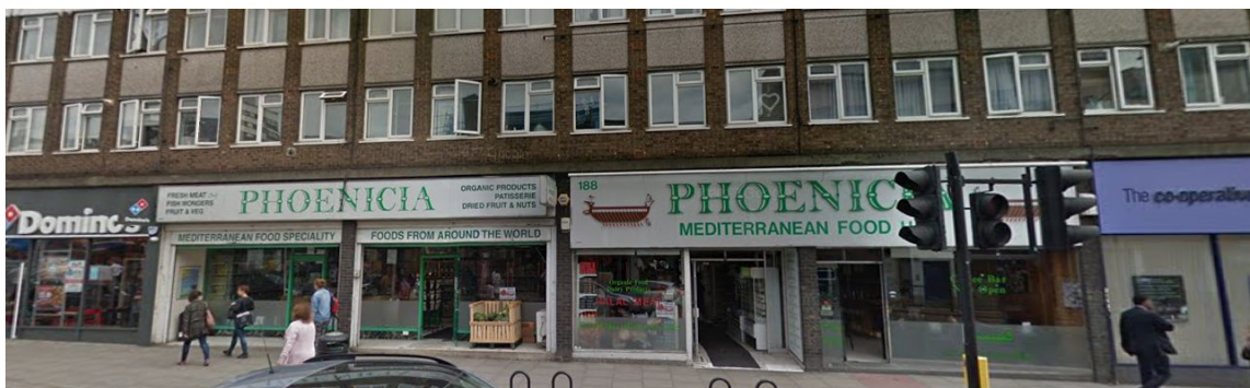
186 -192 KTR, London NW5 2AE Installation of a new shopfront. ref: 26132
