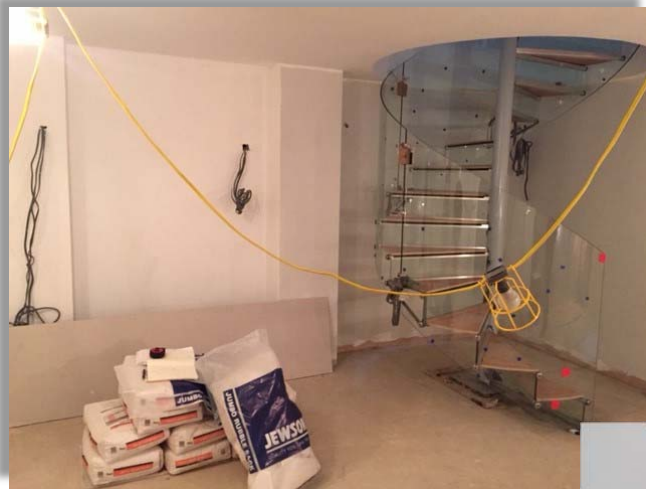
Picture was taken of the basement towards the end of construction.
