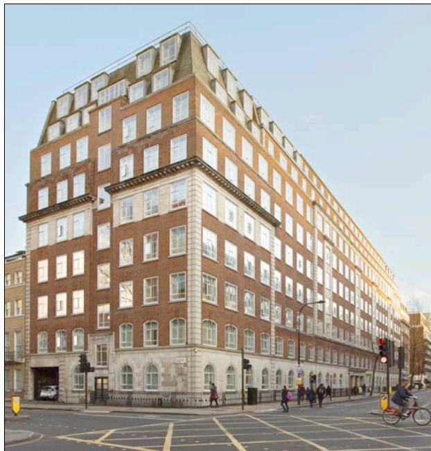
Existing Street View
