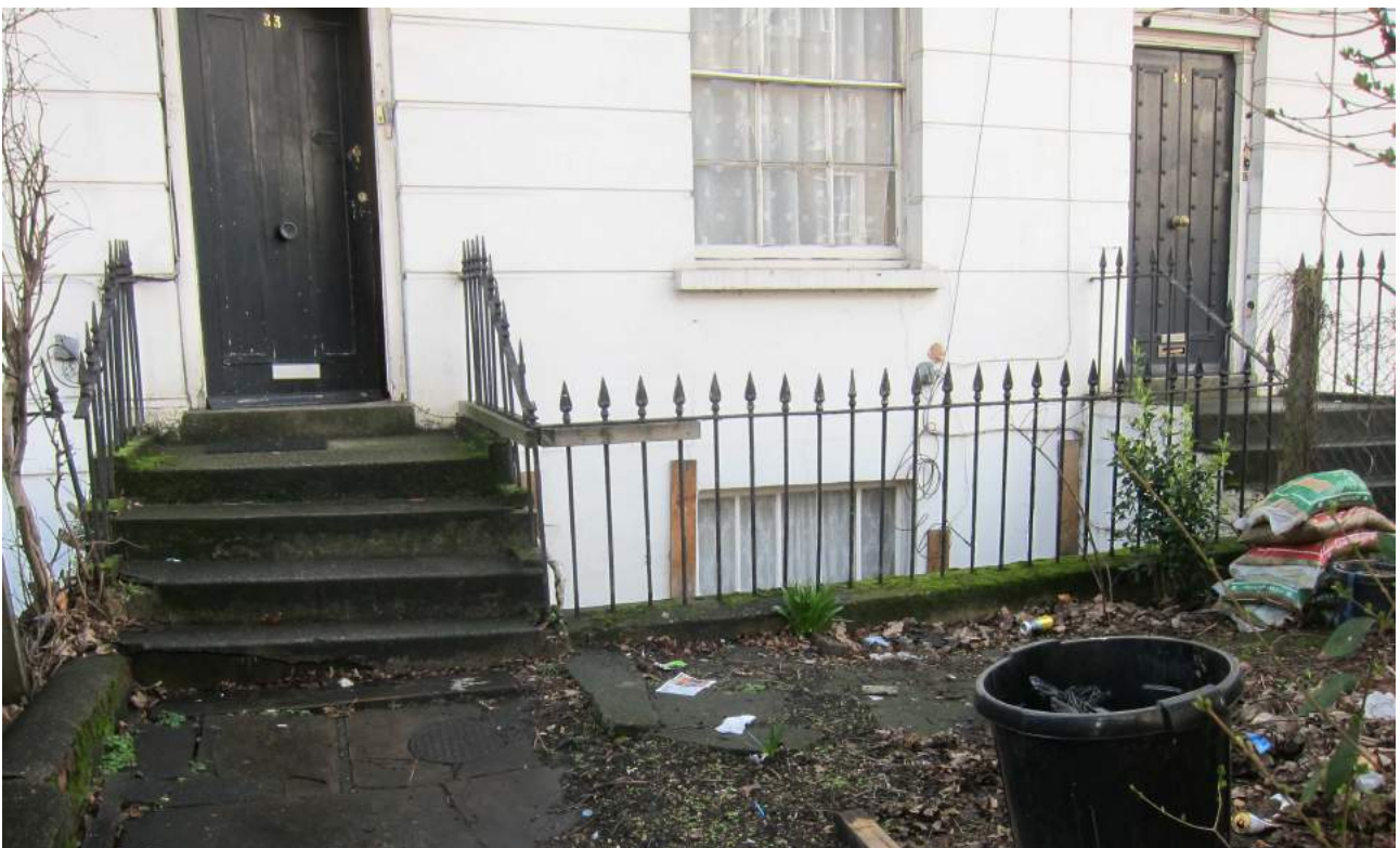
Cast iron railings to front area and entrance steps
