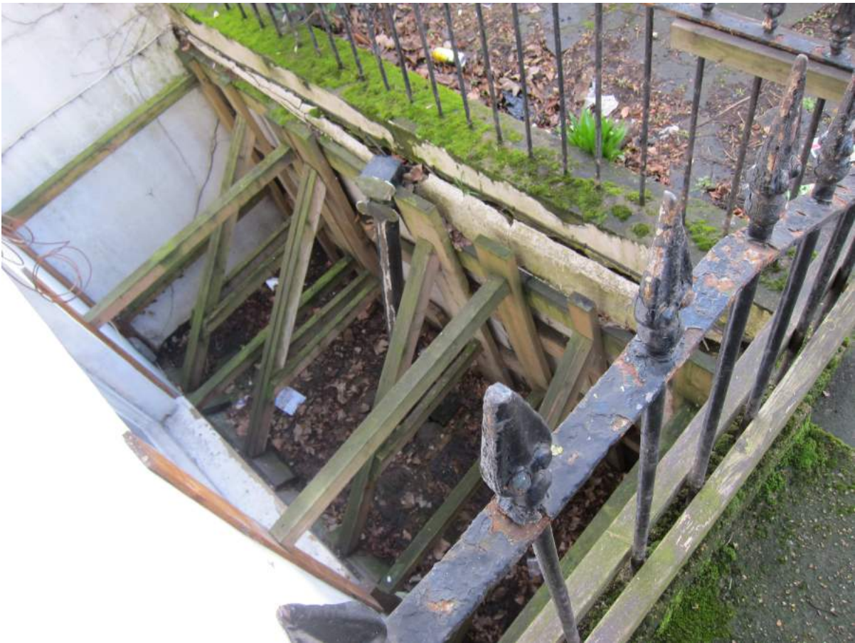
Protective shoring to prevent collapse of front area wall
