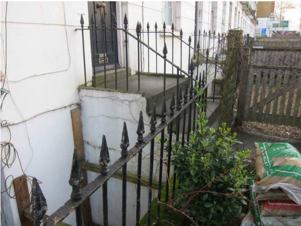
View westwards, with front steps to 35 Crowndale Road in foreground
