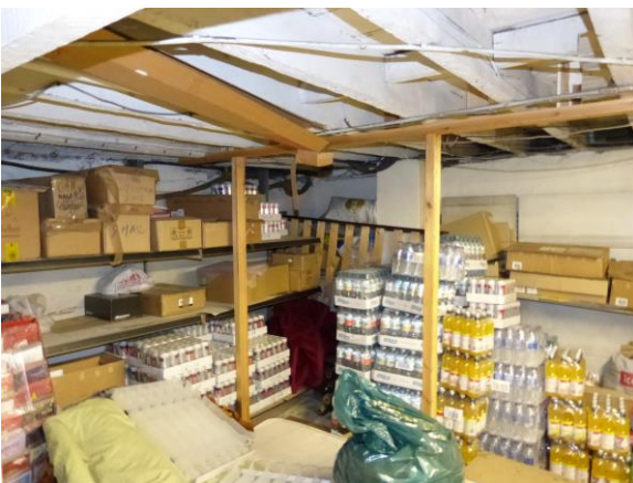
Pic 10 - general view of the basement
