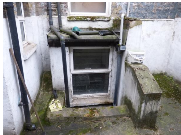
Pic 4 - General view bay projection to be demolished
