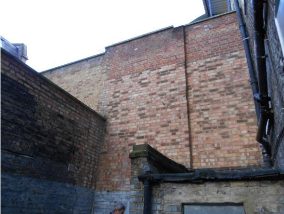
Pic 19 – looking south easterly at courtyard boundary wall
