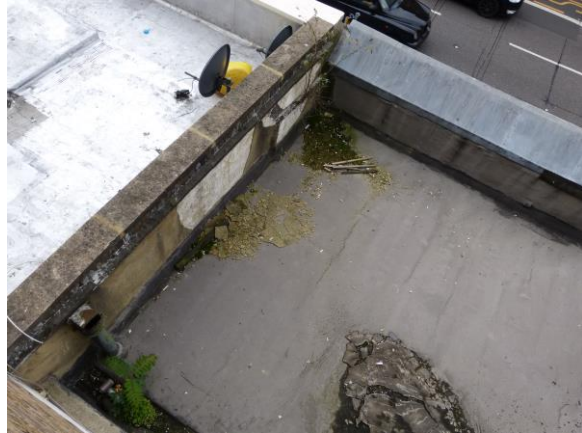
Pic 13 - view of front flat roof
