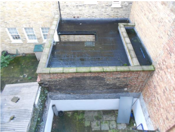
Pic 21 – top floor looking down at rear courtyard
