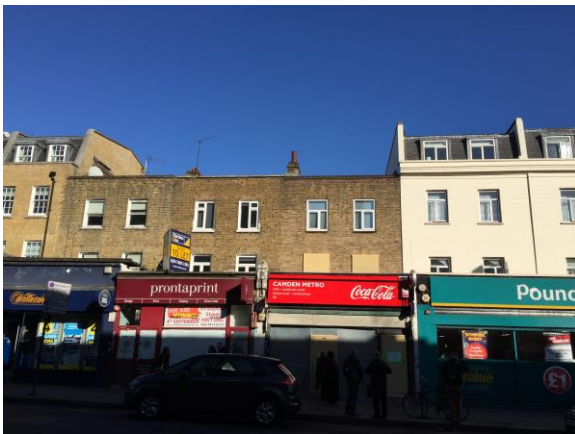
Pic 1.- General view of the west elevation 58 in the centre
