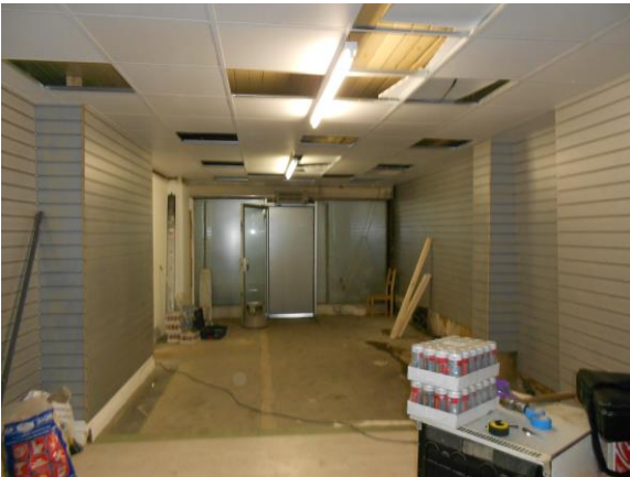
Pic 14 - general view of ground floor shop
