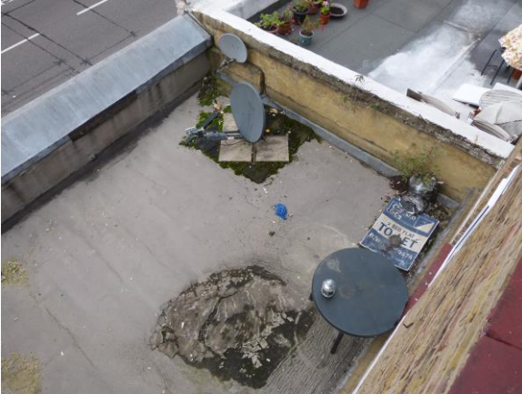
Pic 12 - View from top floor window to front flat roof
