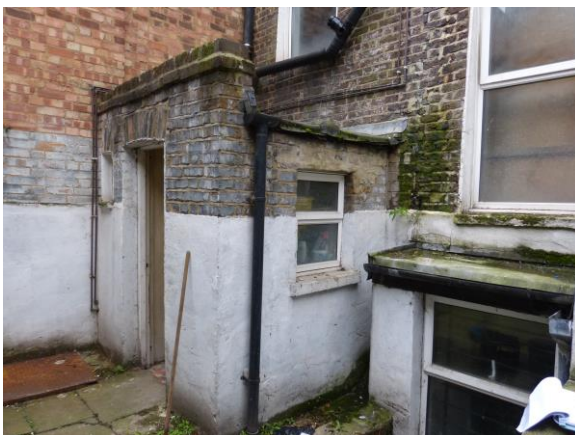
Pic 3 - General view of rear extension to be demolished
