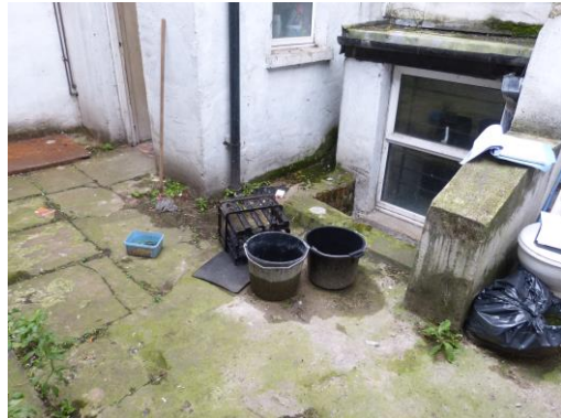
Pic 18 - rear projecting bay and toilet to be demolished
