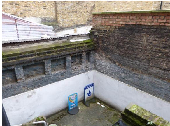
Pic 22 – view of north west boundary wall to courtyard
