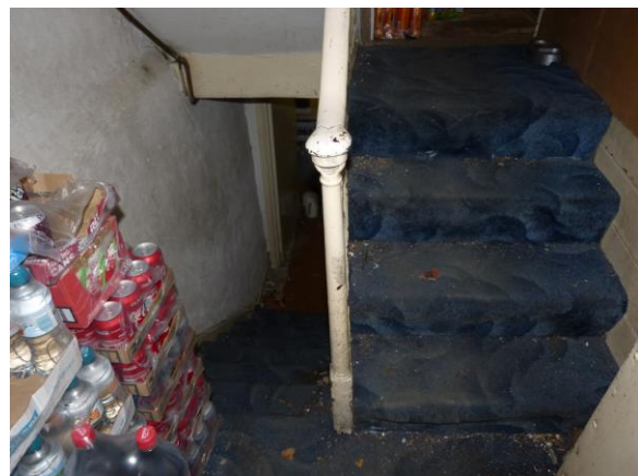
Pic 6 – Upper section of steps to basement
