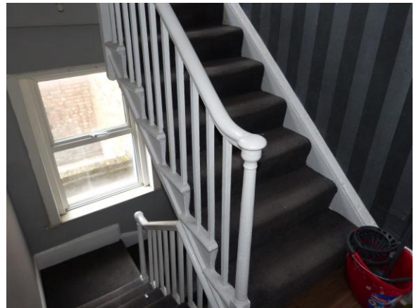
Pic 9 - view from half landing
