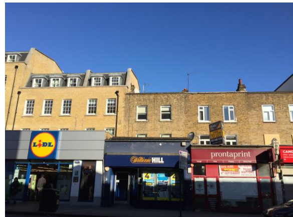
Pic 2 – General view of the west elevation 58 to far right.
