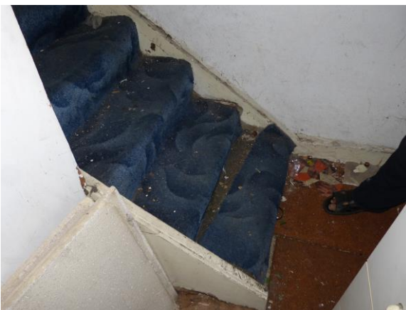
Pic 5 – First section of basement staircase
