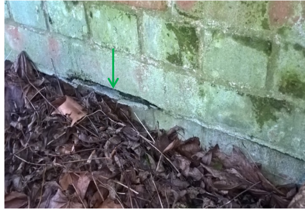
Photograph 6: External – Non-asbestos damp proof course to adjacent external wall.
