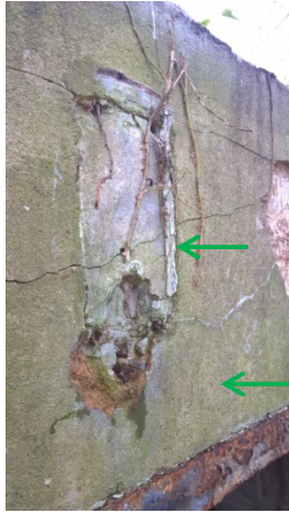
Photograph 5: External – Non-asbestos mastic to former light position. Render to external walls sampled and found to be negative for asbestos.
