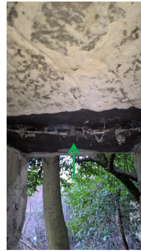
Photograph 2: Ground Floor – G.01 Oil Store – Non-asbestos slate shuttering to vents and windows.
