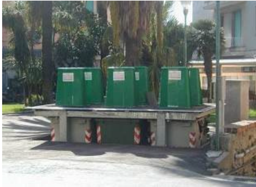
Example of concealed storage on a hydraulic lifting mechanism
