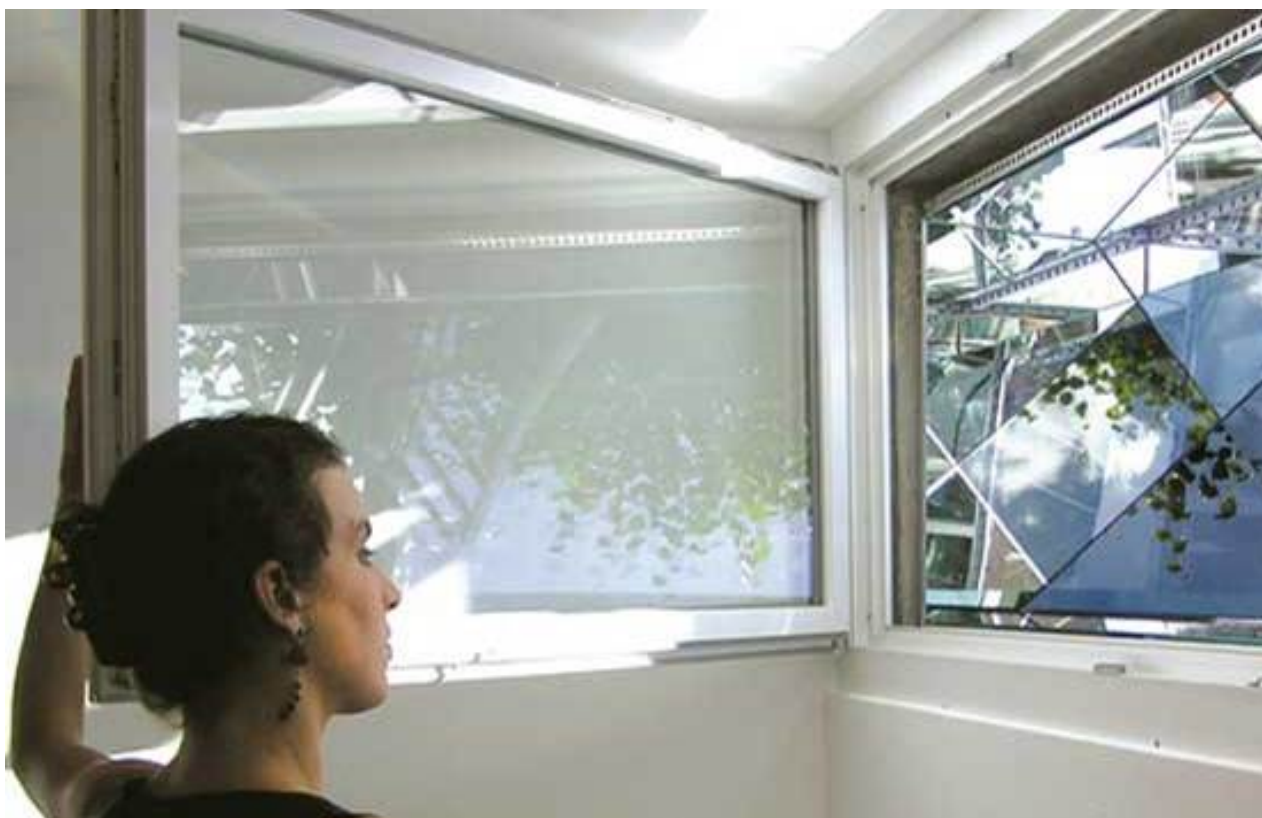
Image of Mirror Shaft technology with obscured glazing panel and objects in front.
