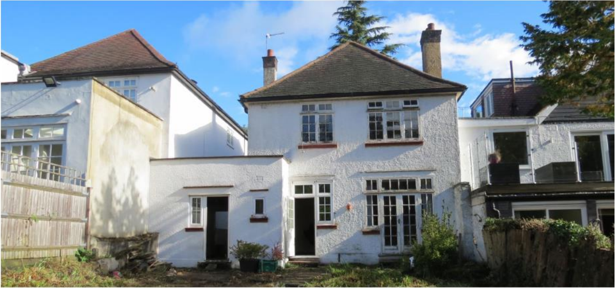
Image 1. Existing rear elevation looking east
