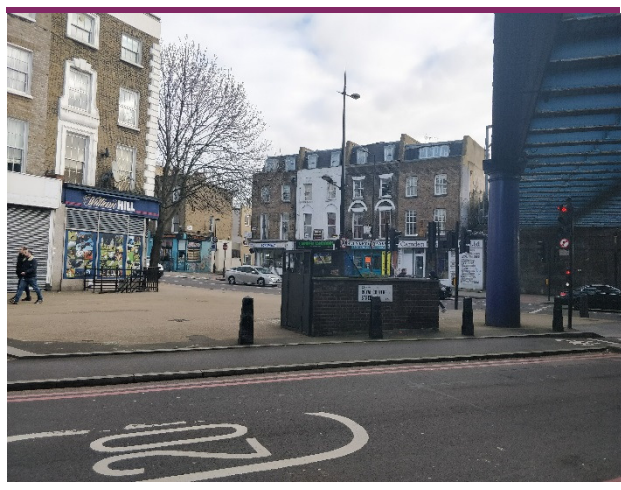
Image 2: View of the Site Looking East
