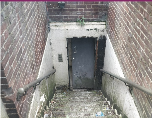
Image 3: View of the Steps as Existing
