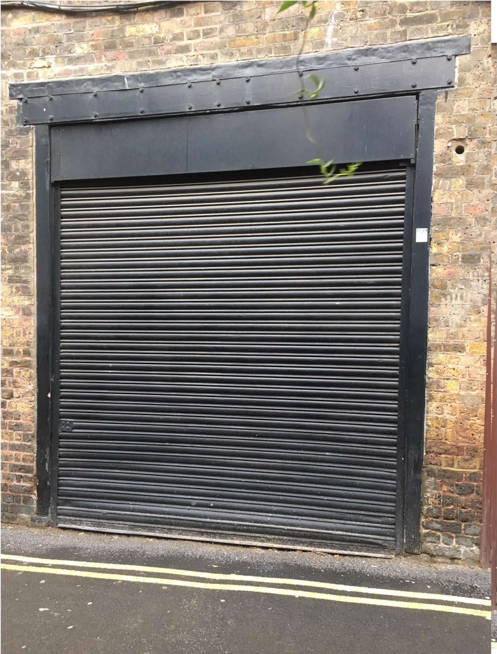
Existing Shutter- closed
