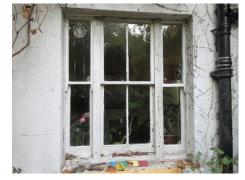
There are a number of single glazed steel Crittall style windows in the property which are not contemporary with the original design and construction. It is not proposed to change the structural openings, but it is proposed to replace these steel windows with painted double-glazed windows to a similar style to the existing.
