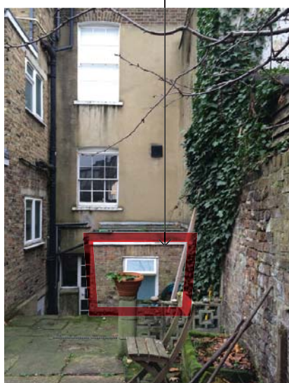
Existing rear elevation showing lean-to bathroom extension to be demolished.
