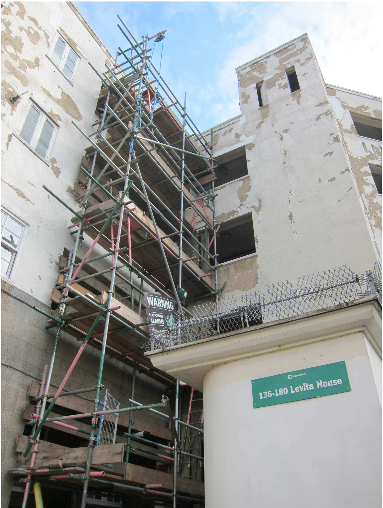
View from courtyard, with scaffolding to protect against falling debris
