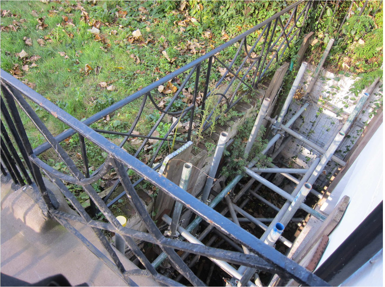
Protective shoring to prevent collapse
