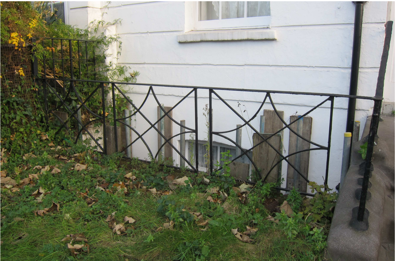
Cast iron railings to front area
