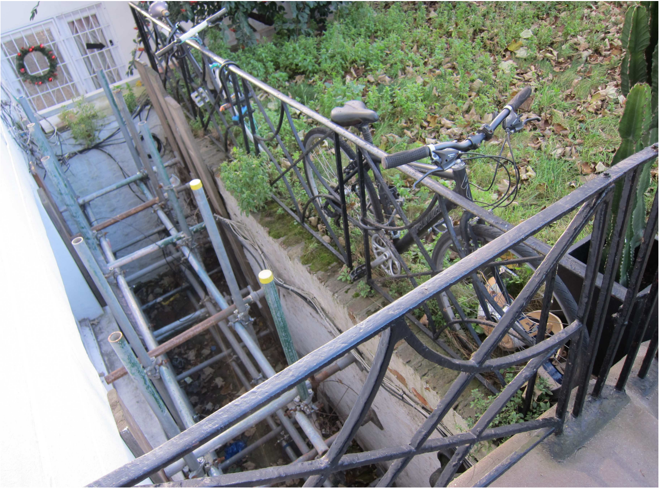
Protective shoring to prevent collapse
