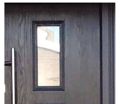
Painted timber door with glazing slot. RAL 7016
