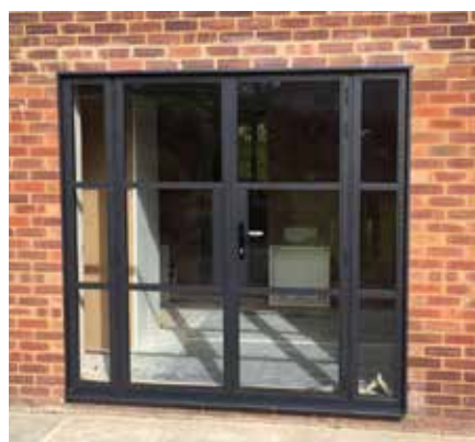
Steel frame windows and doors. Crittall profile. RAL 7016
