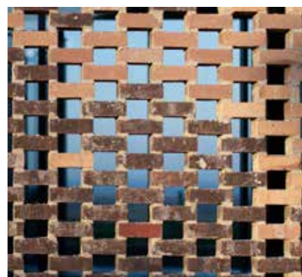
Perforated brick patterning at first floor
